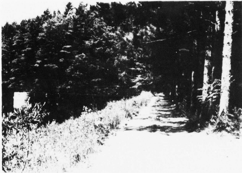
FIGURE 1 CREST OF DAM LOOKING LEFT
