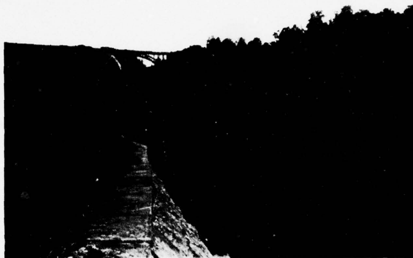
9. View of emergency spillway from stilling basin area. Notice significant vegetative growth in spillway. Left is fence. Discharge tunnel is submerged in basin.
