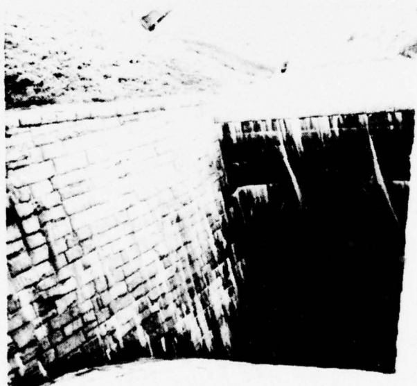
12. View of entrance to discharge tunnel. Some spalling has occurred.
