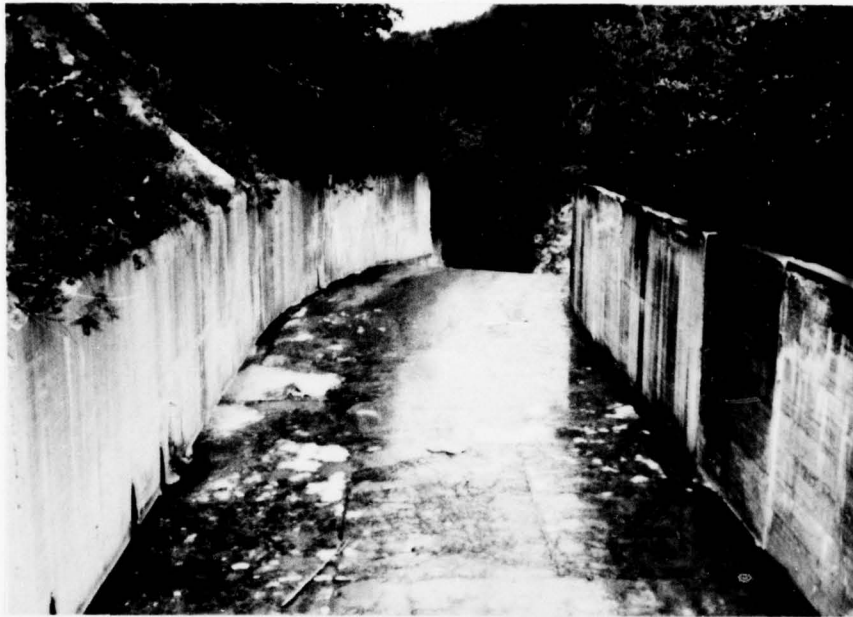
SPILLWAY CHANNEL VIEWED FROM GATE BRIDGE
