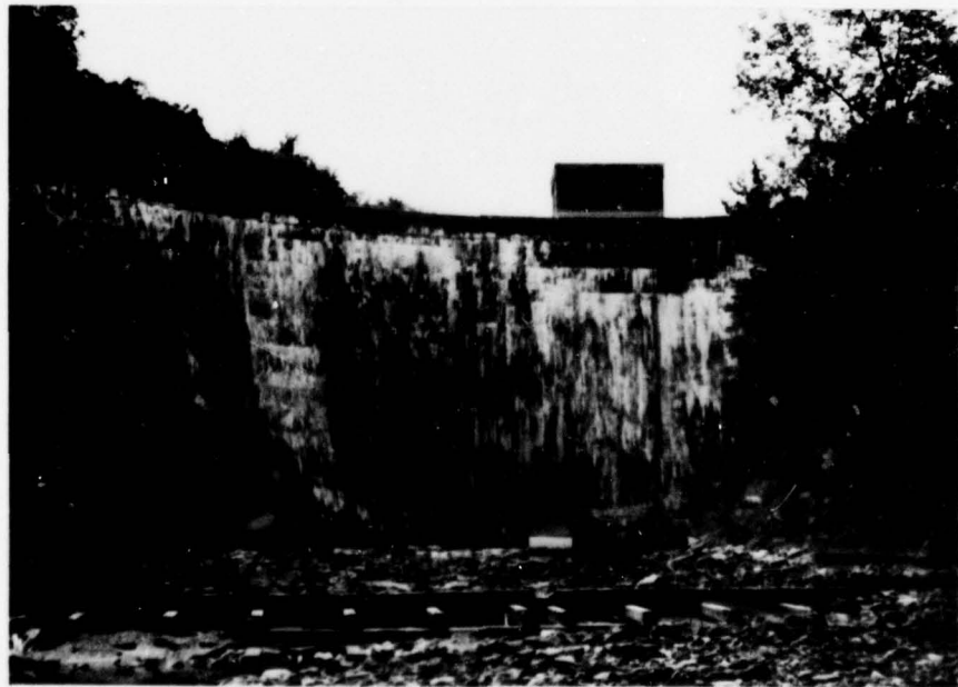
DOWNSTREAM FACE OF DAM FROM DOWNSTREAM WEIR IN STREAM BED
