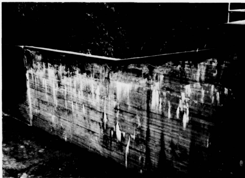
RIGHT WALL, SPILLWAY CHANNEL, FROM GATE BRIDGE
