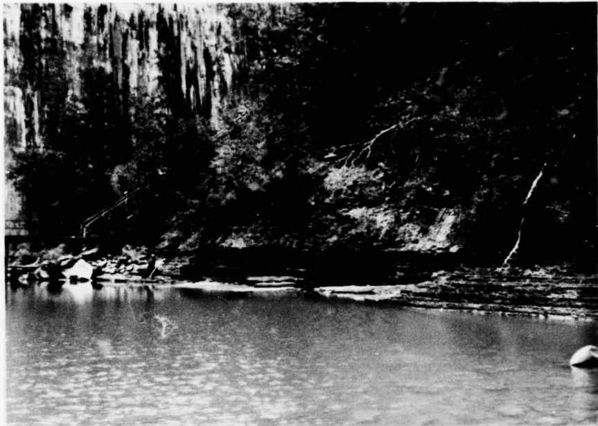
AREA OF SEEPAGE ON LEFT SIDE DOWNSTREAM OF DAM
