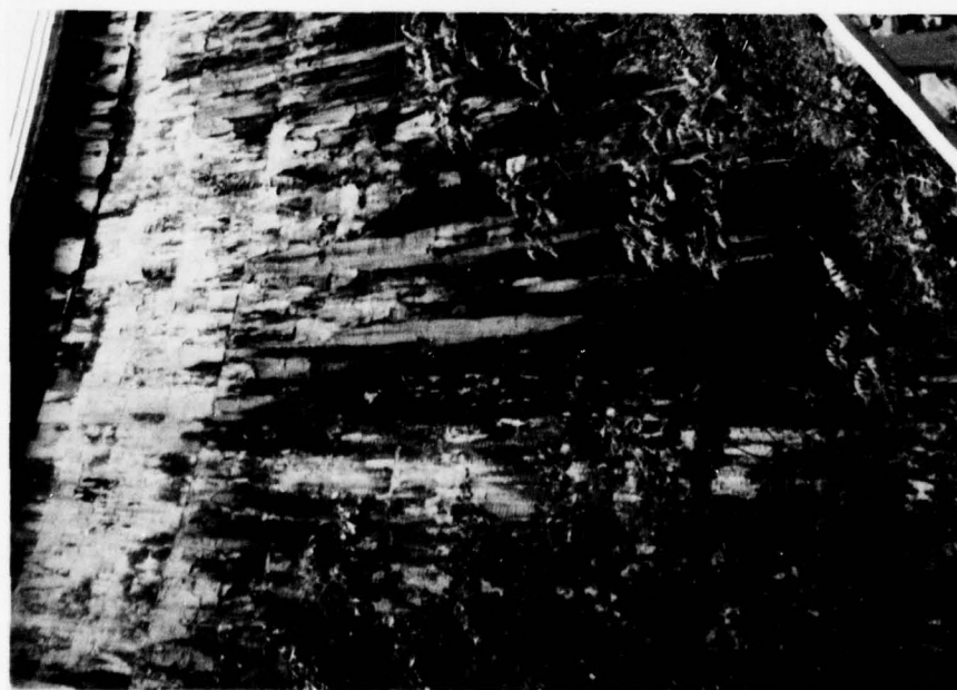
OVERALL VIEW OF DOWNSTREAM FACE OF DAM SHOWING MINERAL DEPOSITION DUE TO SEEPAGE
