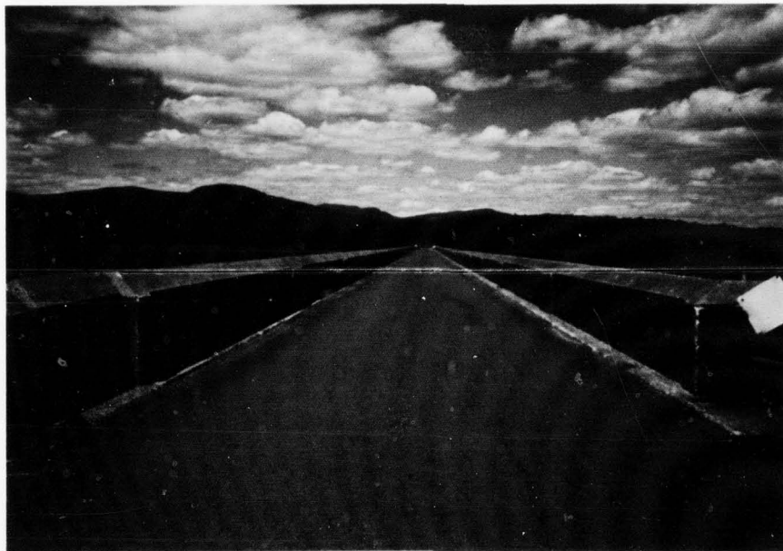
CREST OF OLIVE BRIDGE MASONRY DAM
