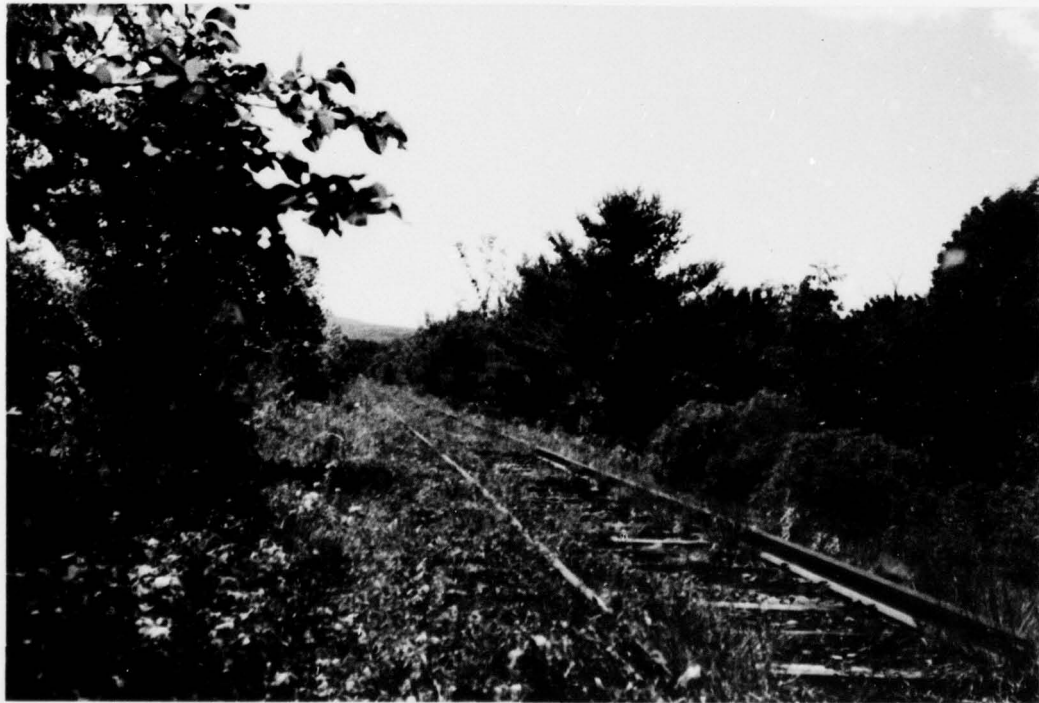
VIEW OF CREST OF GLENFORD DIKE. (LOOKING WEST) NOTE ABANDONED RAILROAD TRACK AND HEAVY VEGETATION
