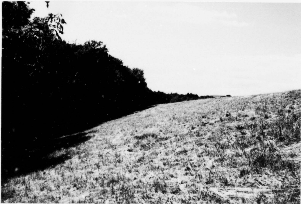
VIEW OF DOWNSTREAM SLOPE OF EAST DIKE. (LOOKING WEST)
