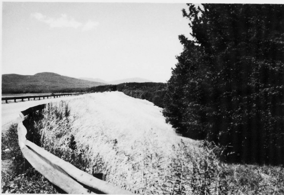
DOWNSTREAM SLOPE OF OLIVE BRIDGE DAM.(LOOKING NORTH)
