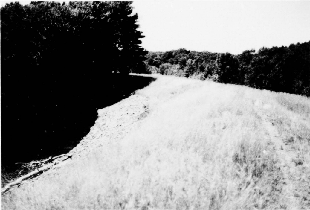
OVERVIEW OF CREST AND UPSTREAM SLOPE OF WOODSTOCK DIKE. (LOOKING WEST) NOTE PATHWAYS AND OVERGROWN GRASS.
