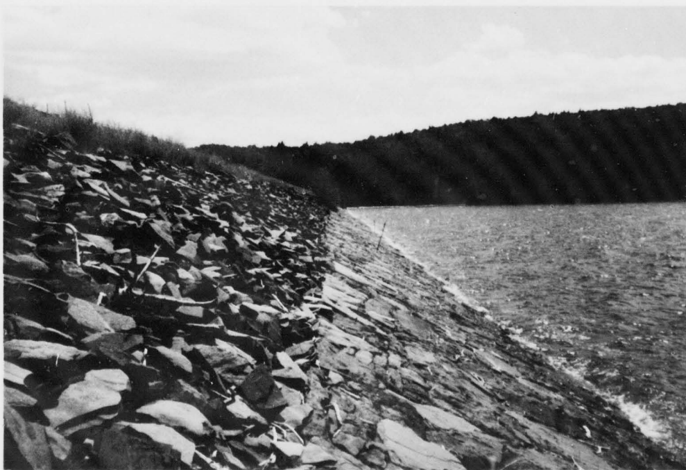
UPSTREAM SLOPE OF SOUTH EMBANKMENT OF DAM.(LOOKING SOUTH)
