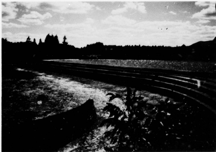
DOWNSTREAM FACE OF SPILLWAY AND FLOOR CHANNEL AND MASONRY WALL. (LOOKING SOUTH)
