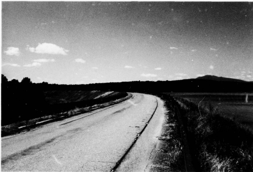
VIEW OF WEST HURLEY DIKE. (LOOKING SOUTH)
