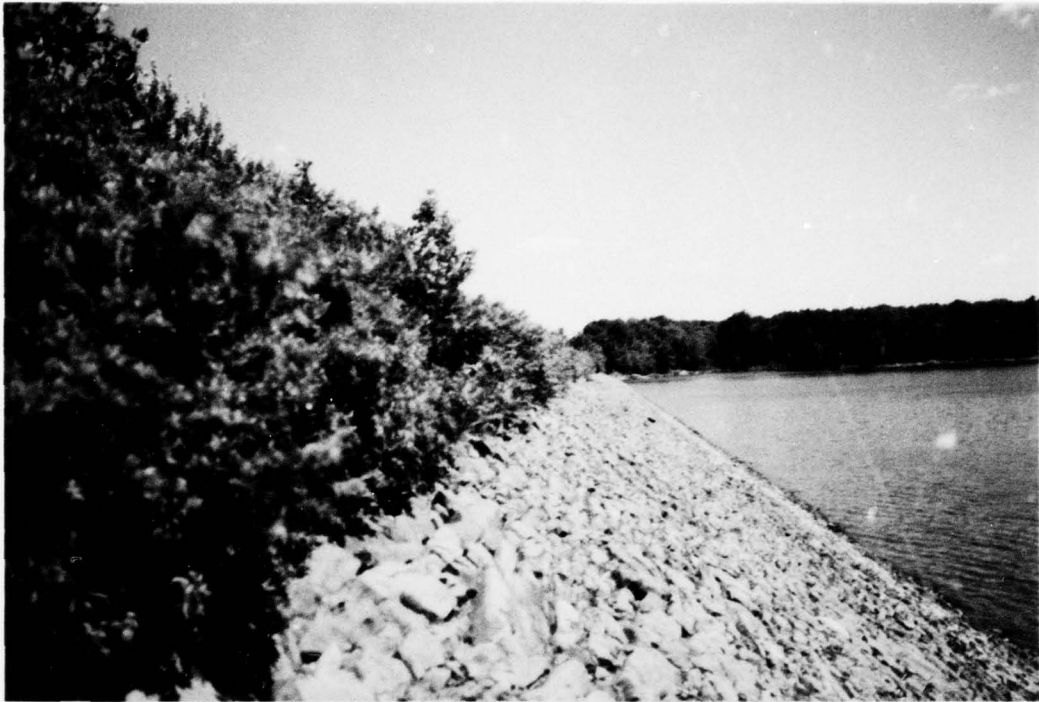
UPSTREAM SLOPE OF GLENFORD DIKE. (LOOKING EAST) NOTE RIPRAP AND HEAVY VEGETATION.
