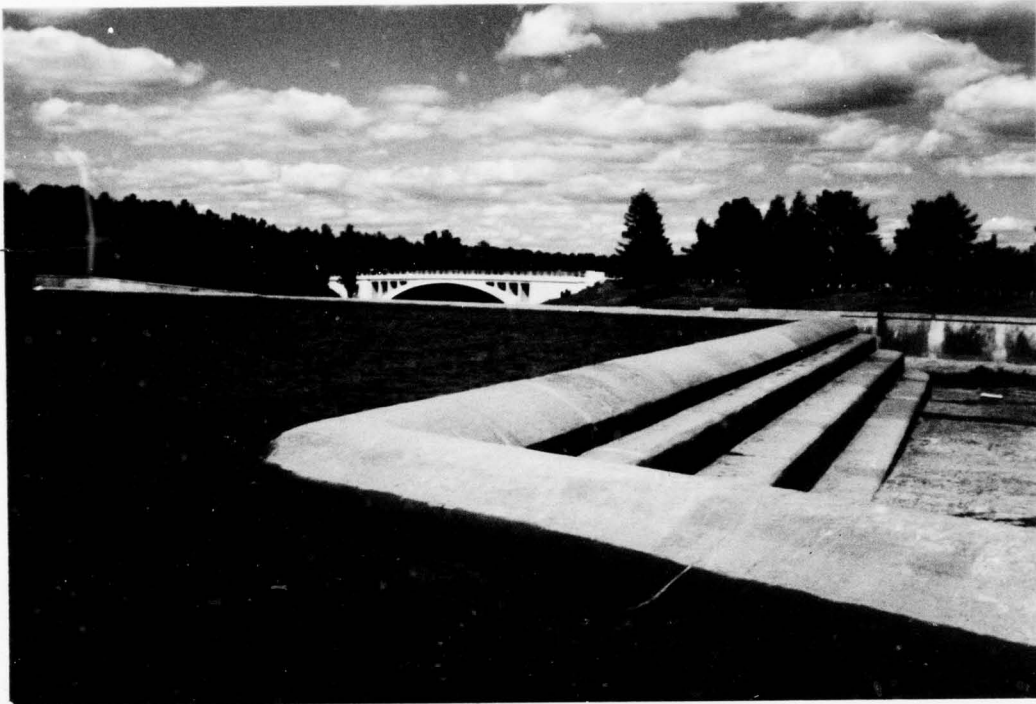
OVERVIEW OF SPILLWAY CREST AND RESERVOIR. (LOOKING NORTH) NOTE MINOR VEGETATION.
