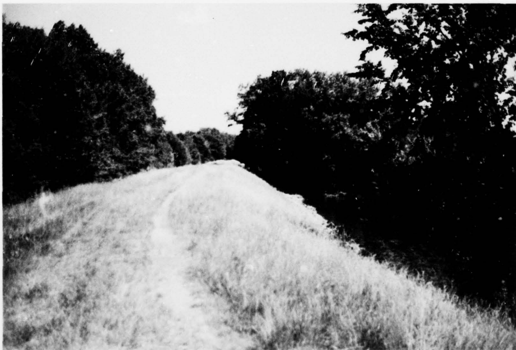
OVERVIEW OF CREST AND UPSTREAM SLOPE OF WOODSTOCK DIKE . (LOOKING EAST) NOTE PATHWAYS AND OVERGROWN GRASS.
