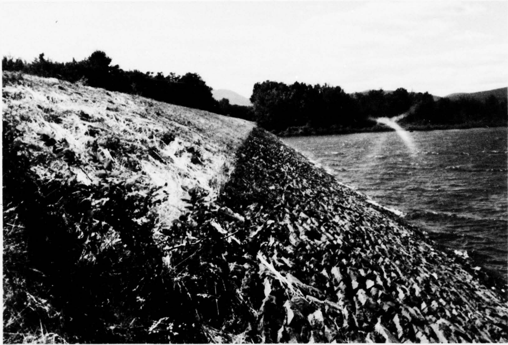
VIEW OF UPSTREAM SLOPE OF EAST DIKE. (LOOKING WEST)
