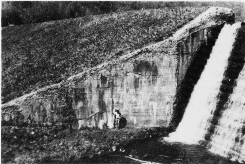
D. Right Spillway Wall
