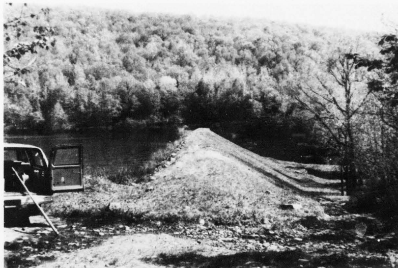
A. Embankment Looking from Right Abutment
