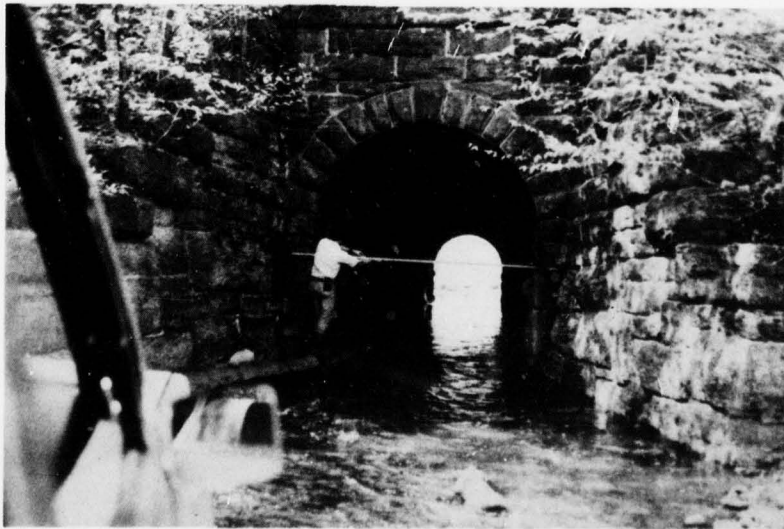
J. Outlet Channel Conduit under Lehigh Valley Railroad located immediately downstream of the Pennsylvania Turnpike Conduit
