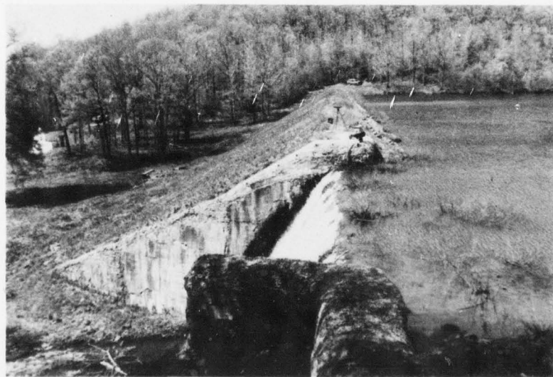
B. Spillway and Embankment Looking from Left Abutment
