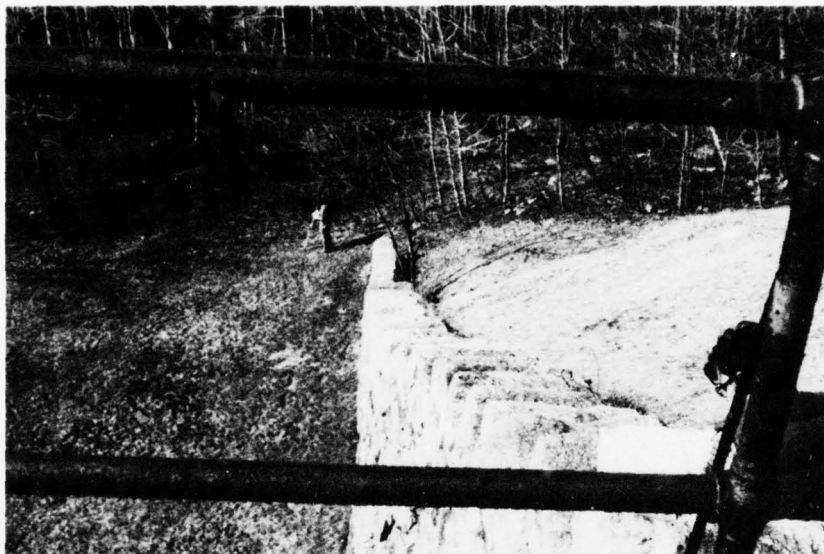
I. Auxiliary Spillway Right Retaining Wall Showing Bow in Wall
