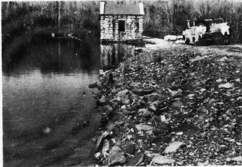
C. Masonry Gate Structure with Right Earth Embankment in Foreground
