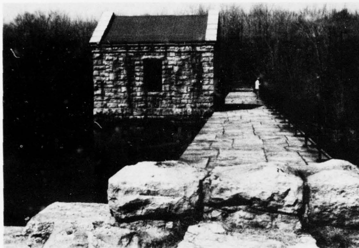
A. Masonry Gate Structure and Auxiliary Spillway
