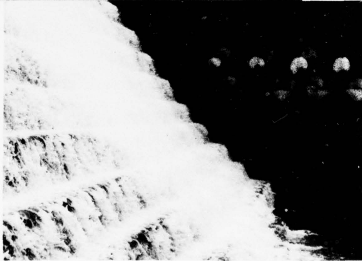
Steps in Spillway
