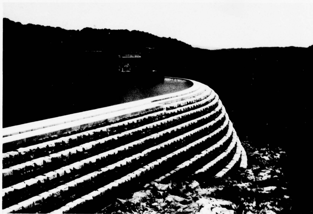
SPILLWAY AND GATE HOUSE NO. 2 (NORTH) VIEWED FROM THE SPILLWAY CHANNEL. THE WATER IN THE CHANNEL IS SEEPAGE FLOW, OBSERVATION (J).
