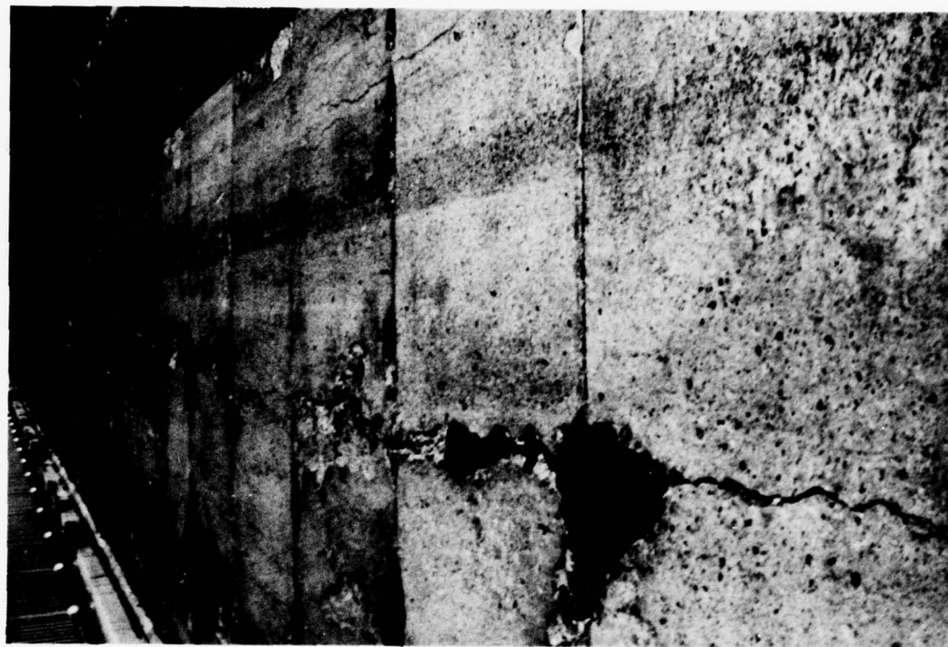
ROAD ON THE CREST OF MASONRY DAM SHOWING CRACKS IN THE PAVEMENT, OBSERVATION (B)
