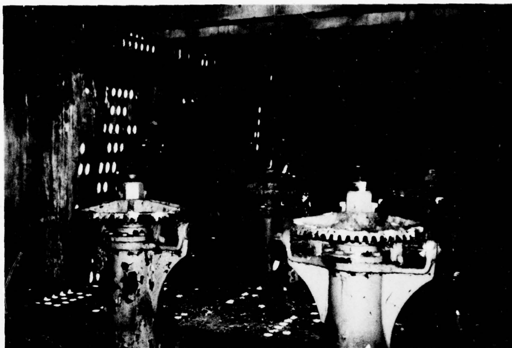
GATE HOUSE NO. 1 (SOUTH) SHOWING RAISED SHIELD AT ENTRANCE TO THE OLD AQUEDUCT LEADING TO THE NEW CROTON GATE HOUSE; MISSING FLOOR PANELS, AND CONDITION OF GATE OPERATING STANDS, OBSERVATIONS (M) AND (P).
