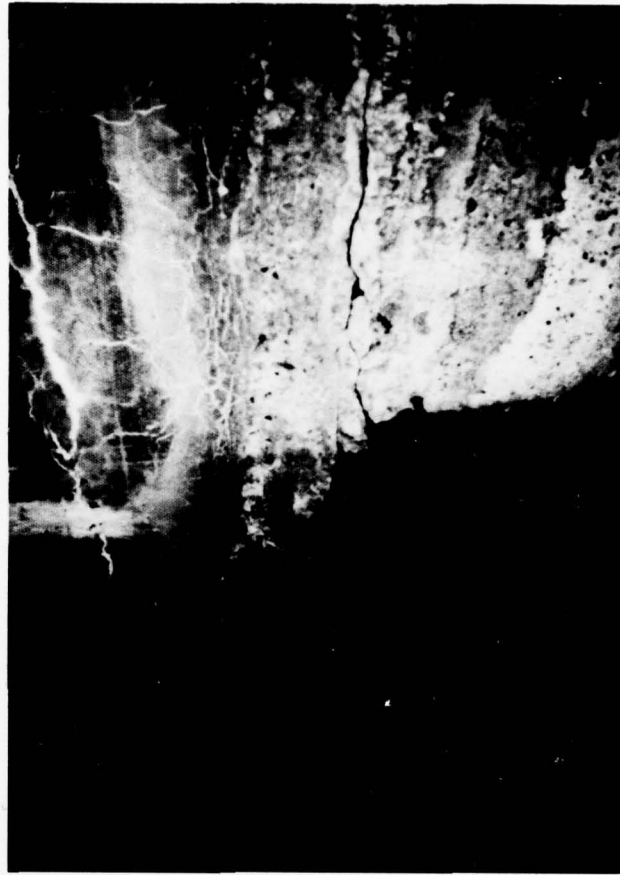
DOWNSTREAM VIEW OF NO. 4 GATE SLOT AREA SHOWING DAMAGED WALL ADJACENT TO ABUTMENT
