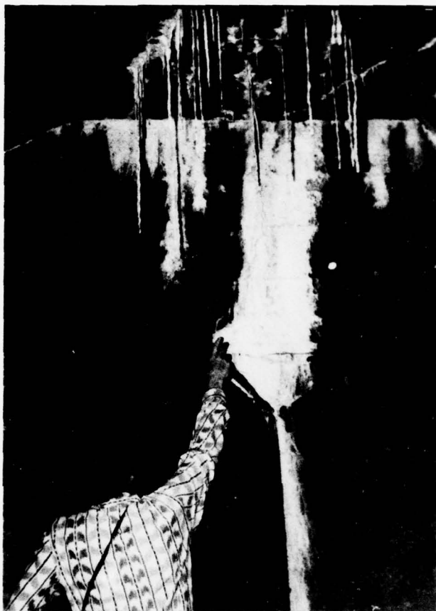
WALKWAY OPENING IN BUTTRESS, SHOWING STALACTITES AND WALL DEPOSITS
