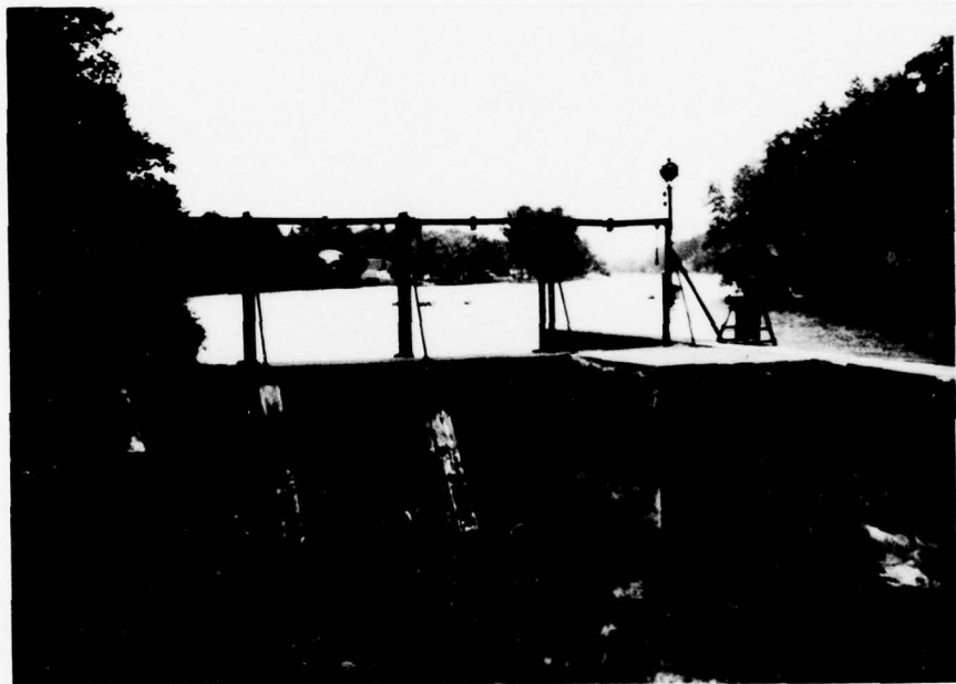
DOWNSTREAM VIEW OF HEAD GATE STRUCTURE ADJACENT TO RIGHT ABUTMENT
