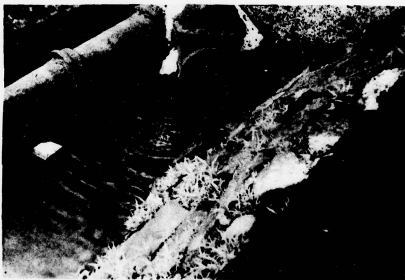
14. Closeup of boil in filtration basin area.
