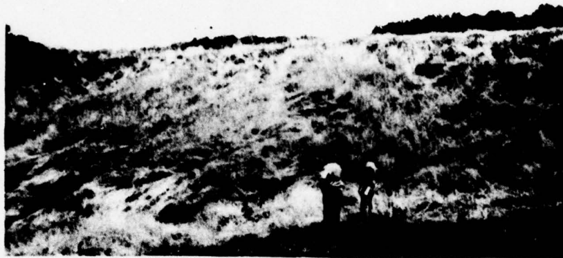
5. View looking north across downstream abutment. Note high grasses. Area being viewed reportedly seeps with high reservoir levels.
