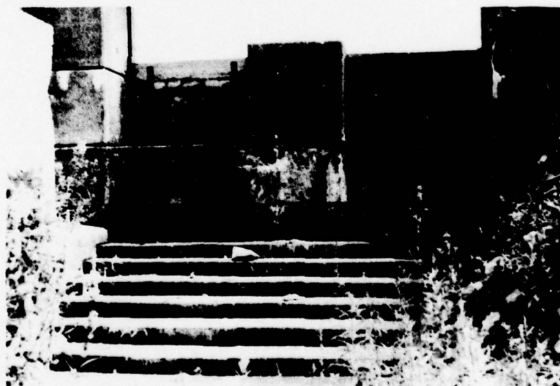
8. Block in center of spillway with damaged spillway sill.
