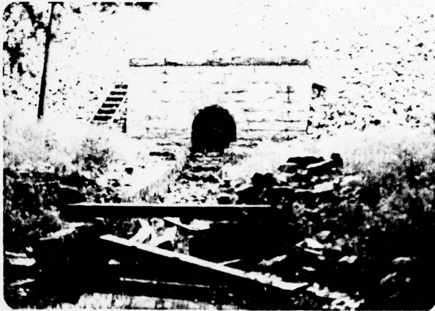
Photograph No. 3 Outlet works.
