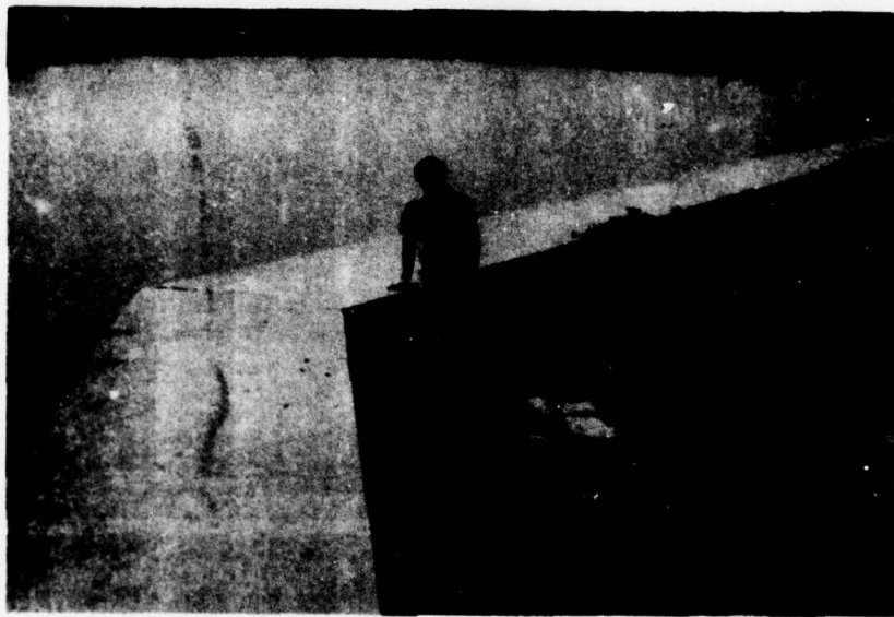
10. Closeup of top of dam showing concrete section on left modification and masonry section on right. Section in between filled with rock. This section has been vandalized, leaving a 2.0-foot hole.
