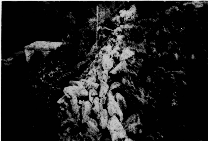
D. Bulges in Riprap on Downstream Slope of Embankment.
