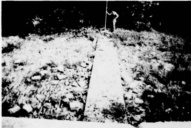
F. Concrete Spillway Weir and Masonry Apron — Flow from Right to Left.
