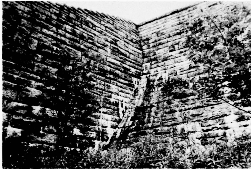
C. Junction of Nonoverflow Section and Retaining Wall
