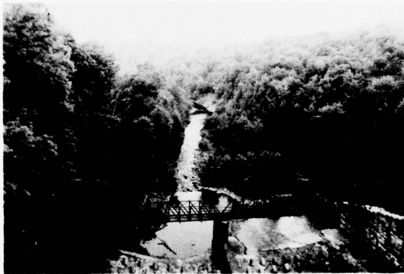
L. View of Downstream Channel from Spillway
