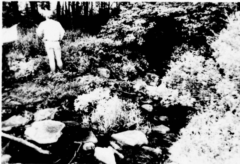
N. Maple Lake Dam — Upstream of Nesbitt Dam — Spillway, View Looking Downstream
