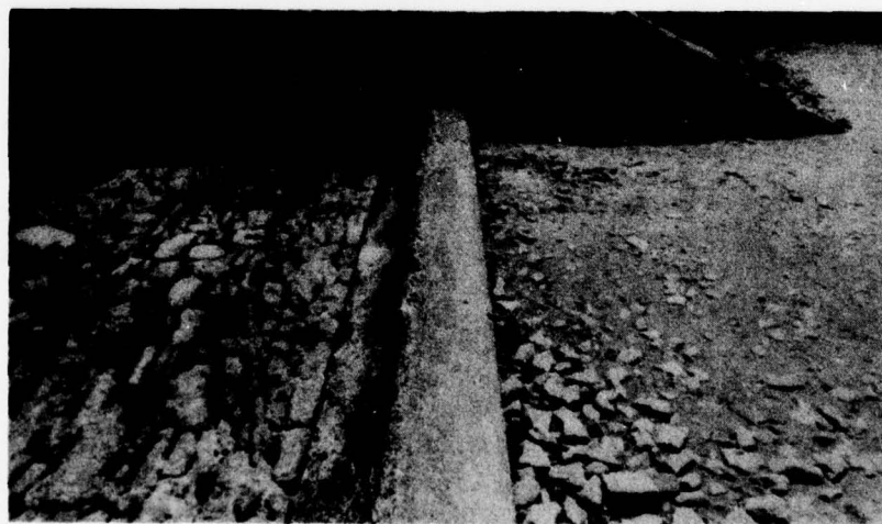
F. Concrete Spillway Weir and Masonry Apron.
