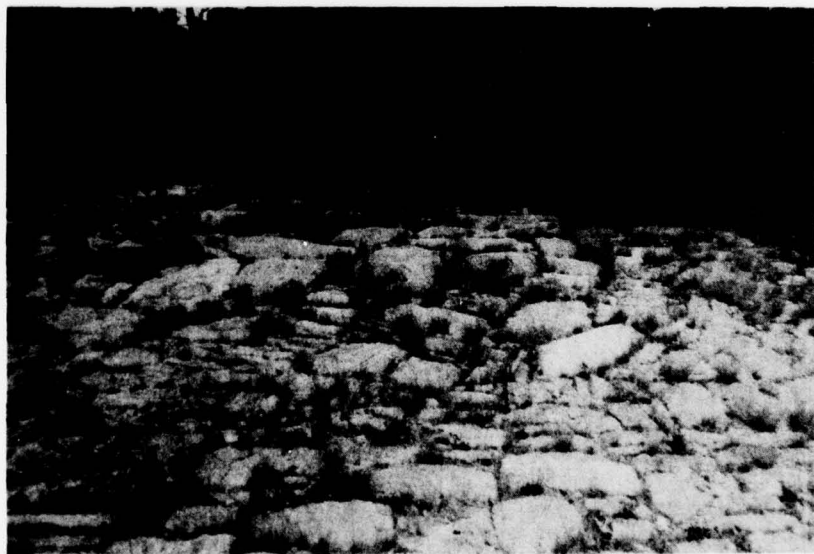
H. Spillway Outlet Channel — Looking Downstream.
