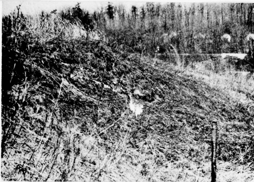
Slide Downstream Slope
