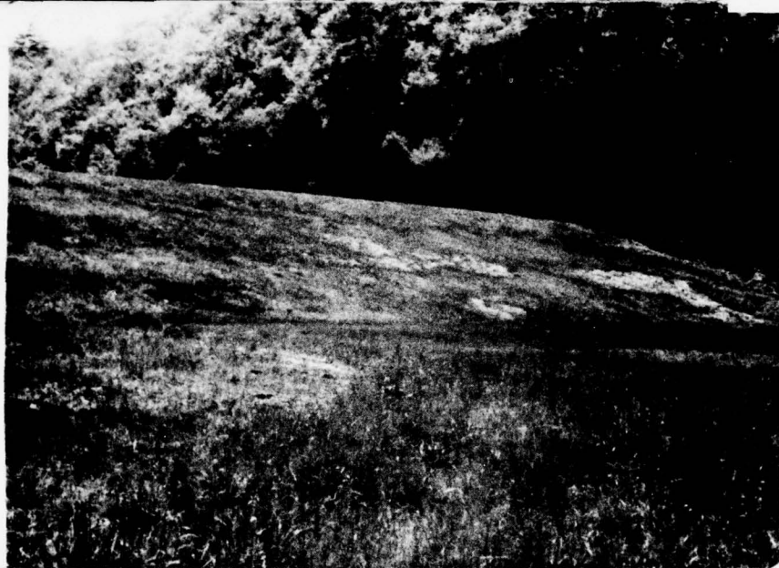
Left Downstream Embankment
