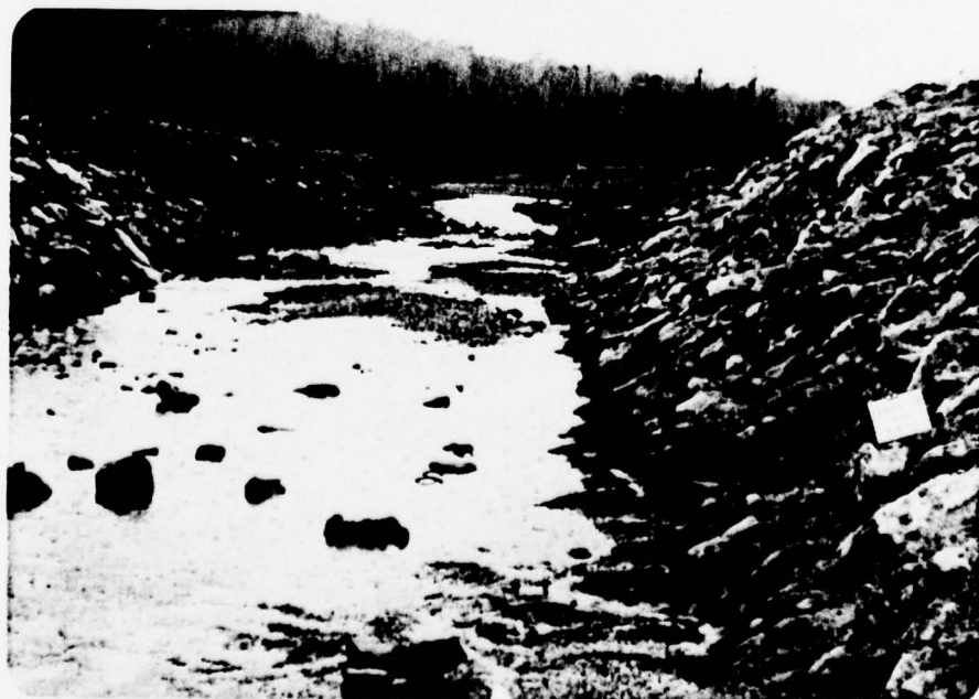
Photograph No. 6 Blow-off pipe plunge pool and discharge channel.
