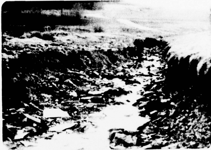
Photograph No. 7 Erosion in discharge channel.
