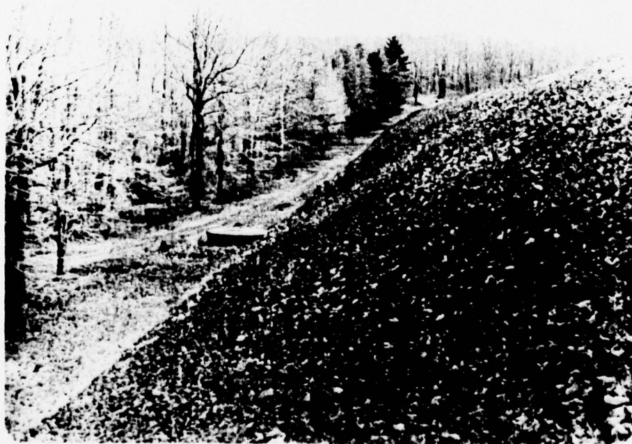
Photograph No. 2 Downstream slope (looking east). Note gate chamber in middle of photograph.
