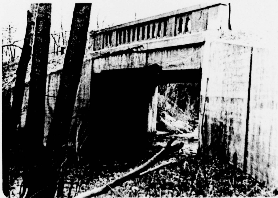
Photograph No. 8 Bridge on Route 711 (Bridge No. 1).
