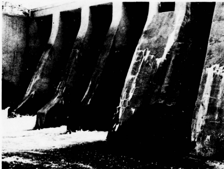
GATE HOUSE PIERS
