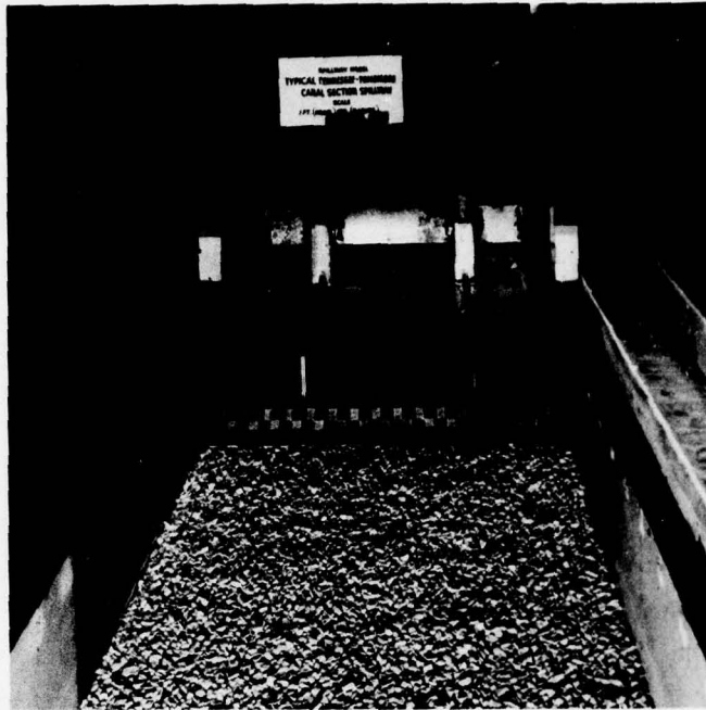
Figure 16. Spillway B, type 3 riprap, type 4 stilling basin, type 2 divider wall
