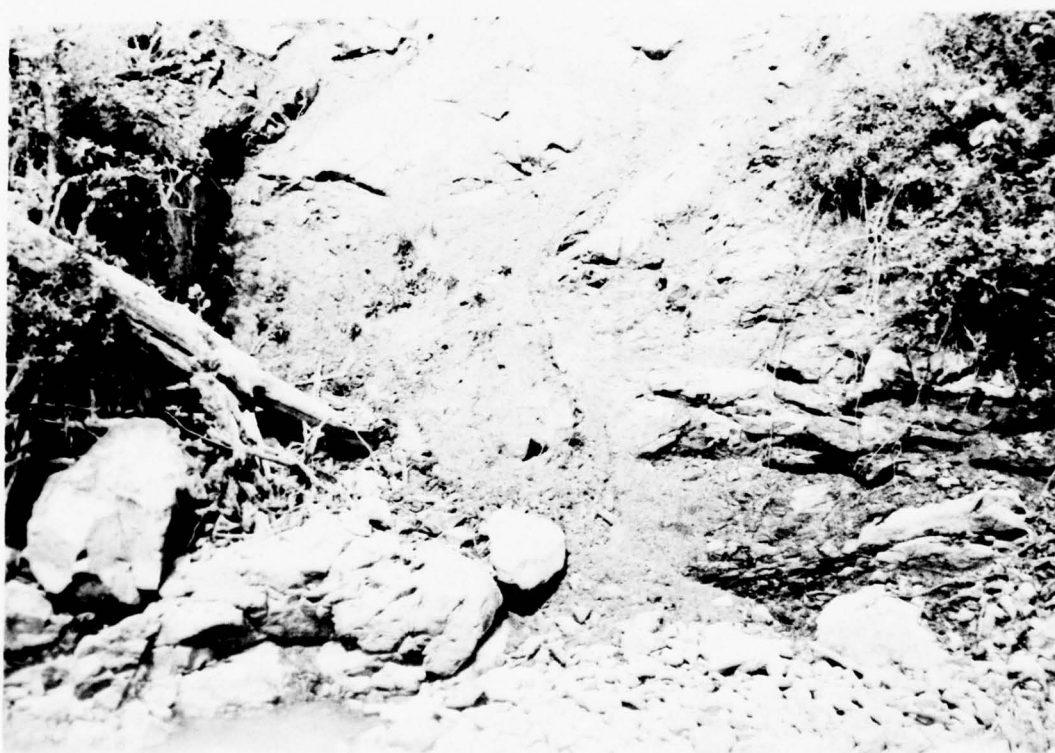
EROSION DOWNSTREAM LEFT ABUTMENT
