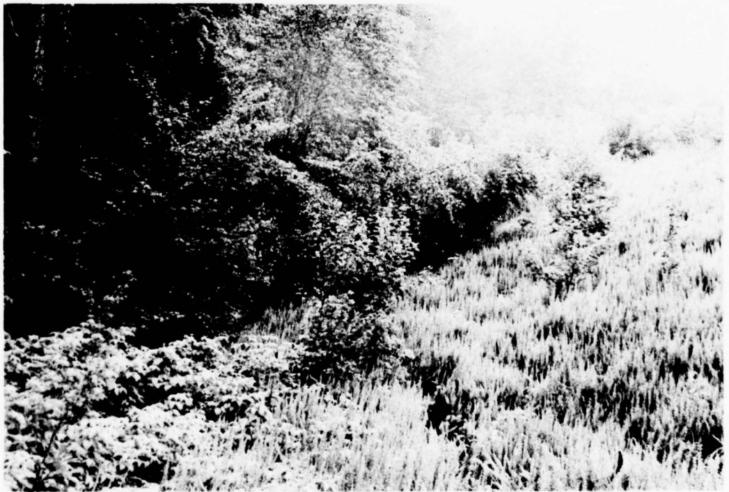
PHOTO 6. Brush and Trees on Downstream Embankment Near Intersection With Right Abutment
