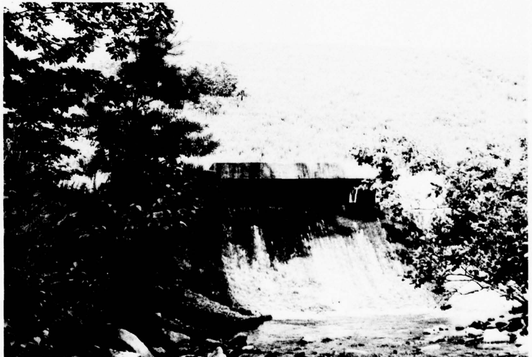
PHOTO 2. View of Outlet Structure Below the Embankment
