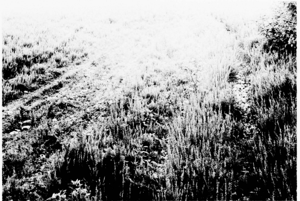
PHOTO 8. Erosion From Vehicle Traffic on Downstream Face Near the Left Abutment
