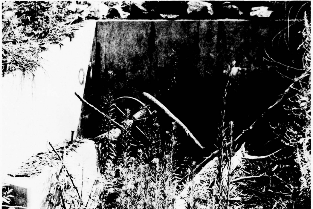
PHOTO 5. Pit for Operational Valves at Base of Front Face of Embankment
