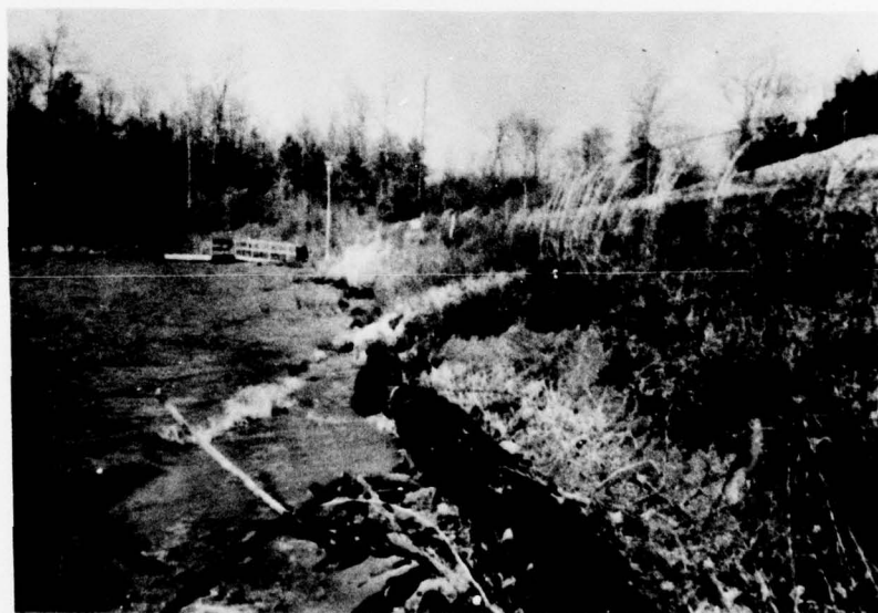
GEORGE F. BRASFIELD - VIEW OF BANK EROSION ON U/S SLOPE OF LEFT ABUTMENT
