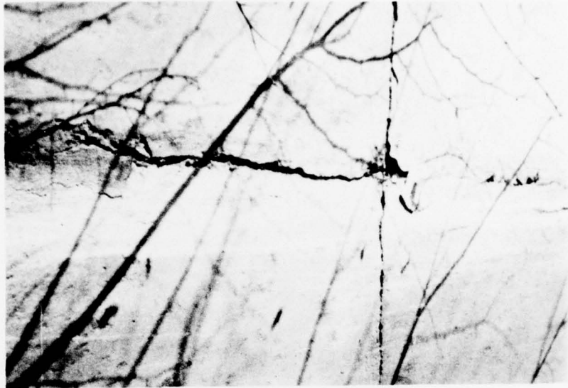
GEORGE F. BRASFIELD - VIEW OF SPALLING ON D/S FACE ALONG JOINTS
