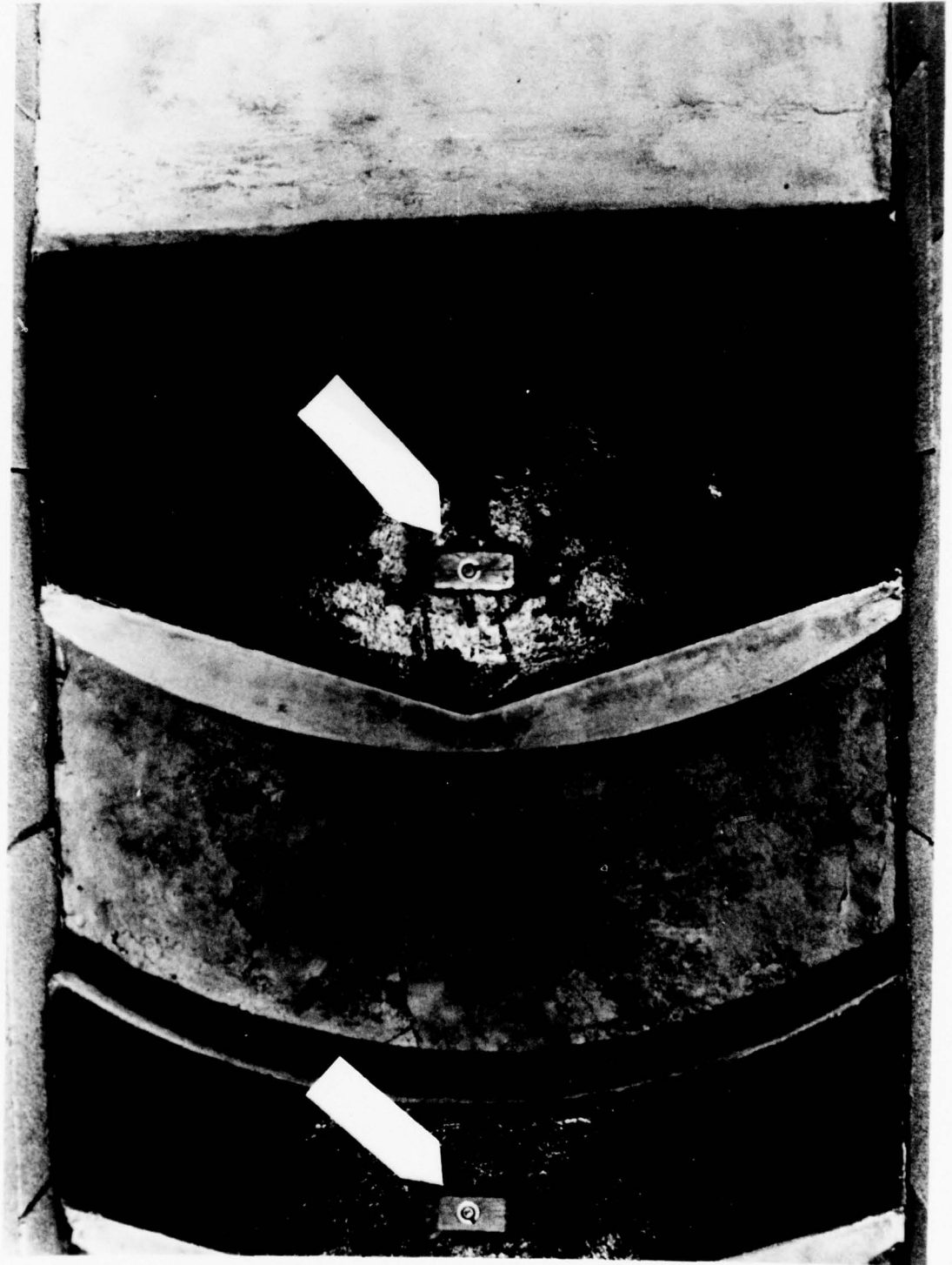
Figure 4 Lock Floor Showing Pressure Gages on Lock Door Sills
