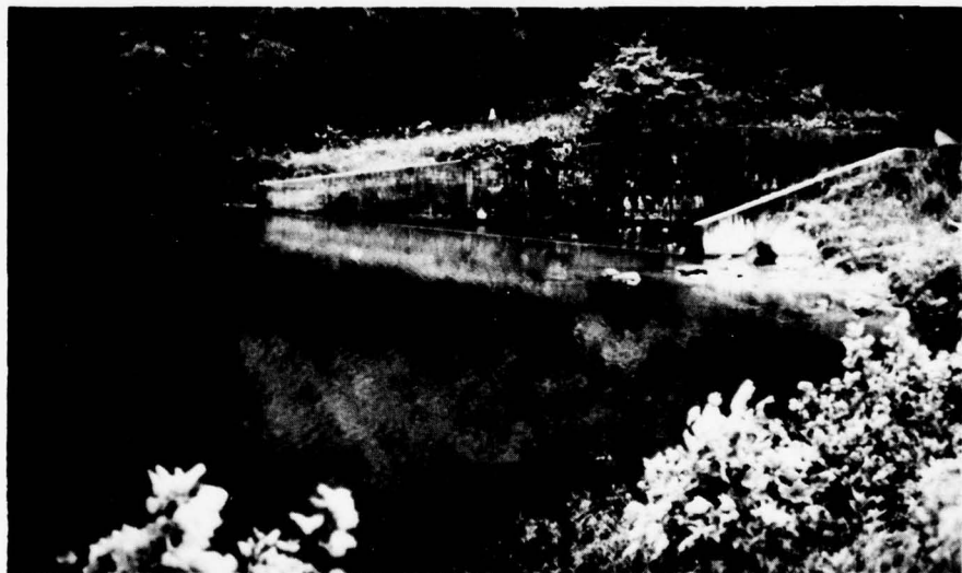
SPILLWAY CREST AND CONCRETE SPILLWAY CHANNEL
