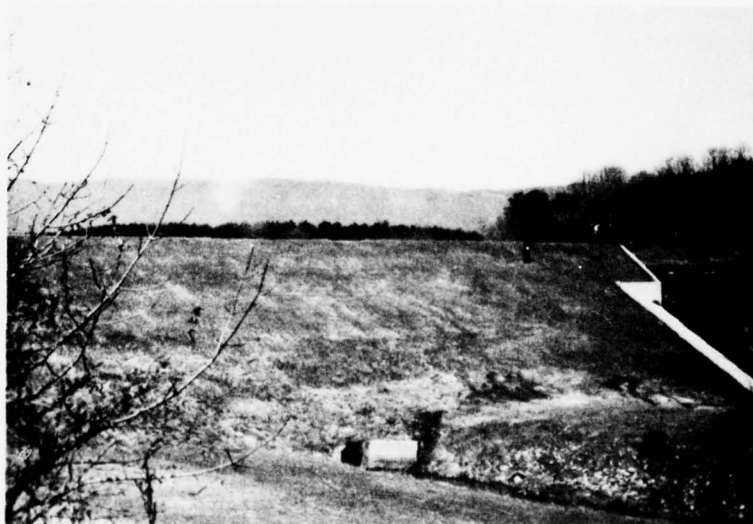
Downstream Slope and Outlet
