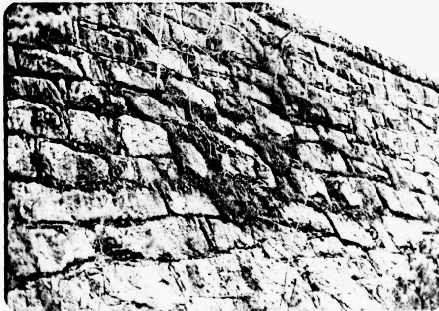
Photograph No. 2 Downstream slope.
