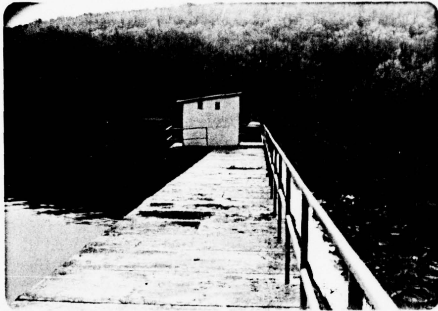
Photograph No. 1 Dam crest.
