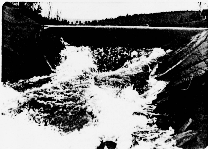
Photograph No. 2 Primary spillway.
