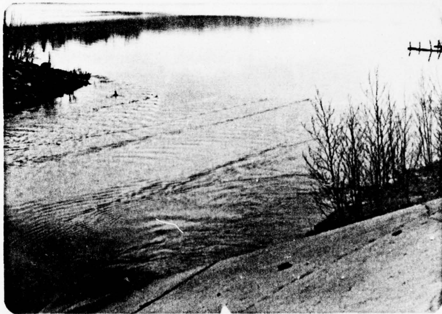
Photograph No. 3 Primary spillway approach channel.
