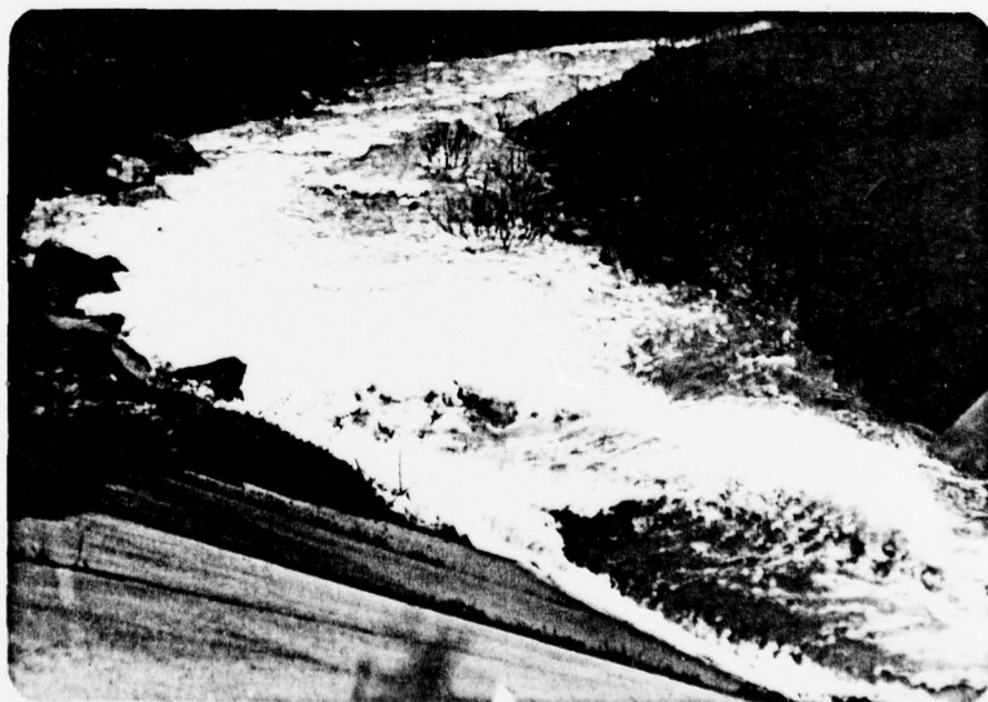
Photograph No. 4 Primary spillway discharge channel.
