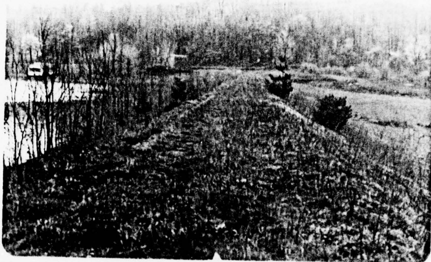
Photograph No. 1 Dam crest.
