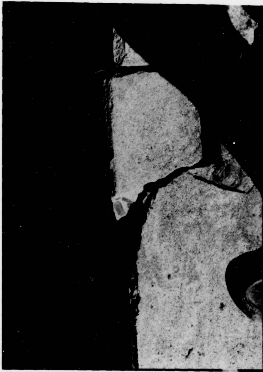
LEFT RETAINING WALL OF EMERGENCY SPILLWAY LOOKING DOWN AT COMPRESSION FAILURE AT CONSTRUCTION JOINT. SPILLWAY CHANNEL IS LOCATED AT TOP OF PHOTO. TWO JOINTS OF THIS NATURE WERE OBSERVED.
