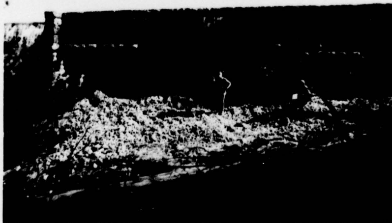
H. Disintegrated Concrete at Downstream Face of Auxiliary Spillway
