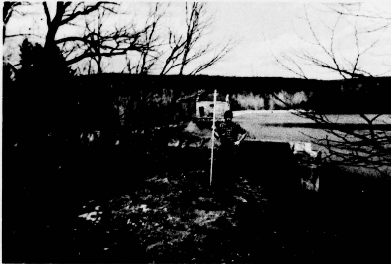
C. Left Approach Wall of Auxiliary Spillway Showing Low Area Behind Wall
