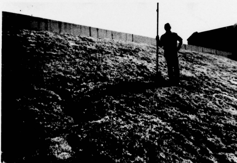
K. 1916 Piezometer and Groundhog Burrowing on Downstream Embankment Surface
