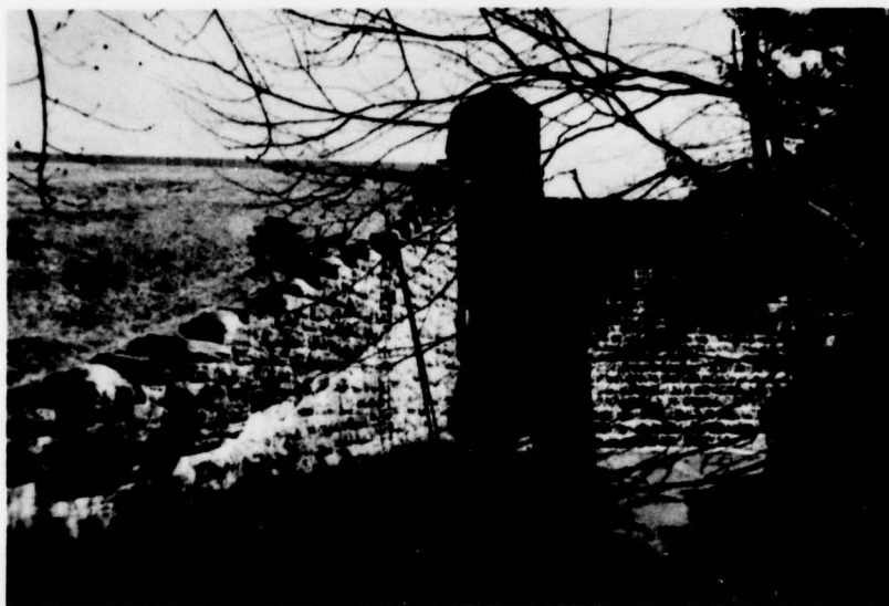
I. Masonry Retaining Wall Between Embankment and Outlet Channel of Main Spillway Showing Repaired Diagonal Crack and Disintegration of Concrete Caps - Wet Area Shown Behind Retaining Wall
