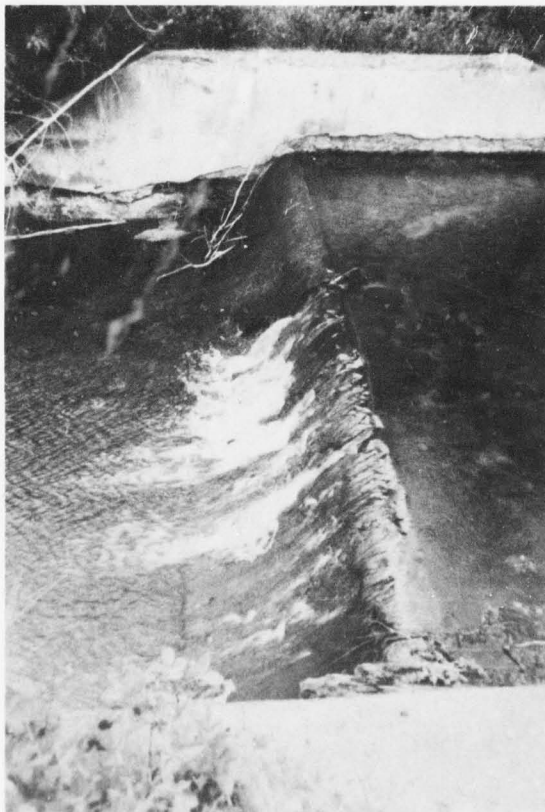
L. Compton Dam — Upstream of Watres Dam — Spillway at Right Abutment of Dam
