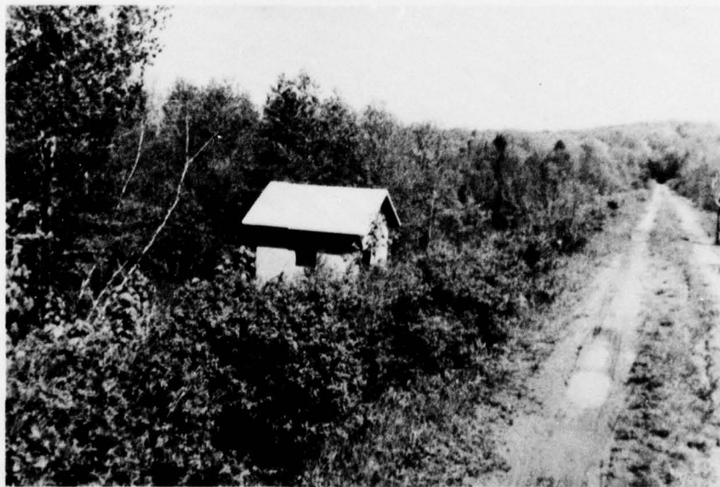
B. Valve House and Top of Dam Looking Towards Right Abutment
