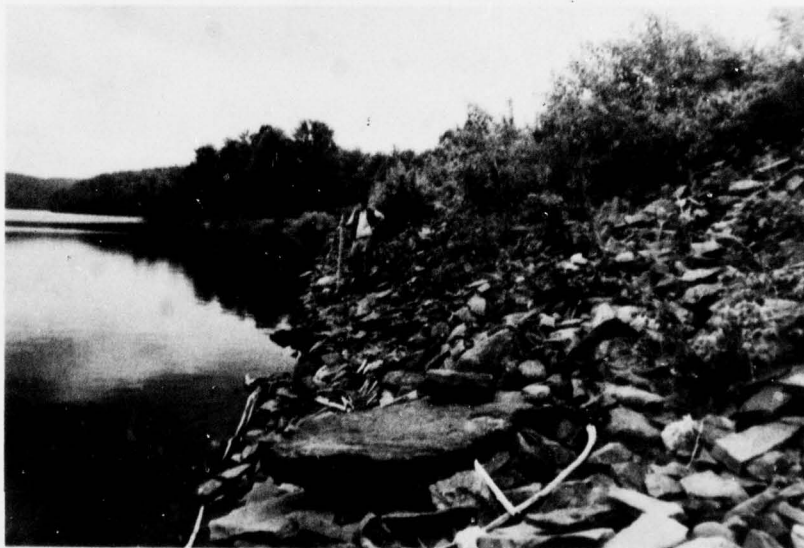
D. Riprap on Upstream Slope of Embankment
