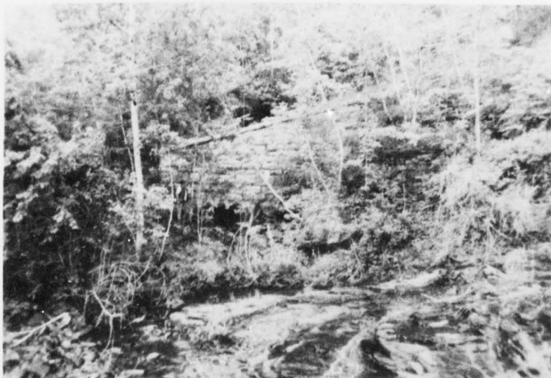
J. Retaining Wall on Right Bank of Downstream End of Spillway Channel
