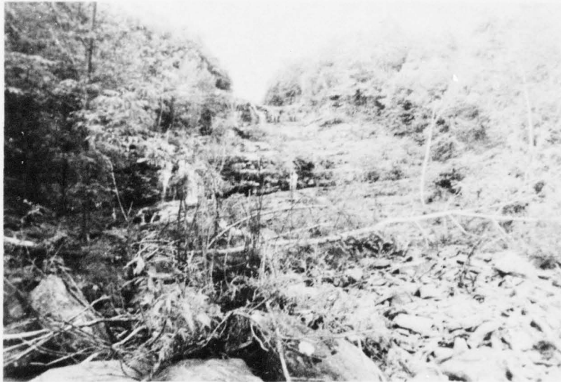
I. Downstream End of Spillway Channel Looking Upstream
