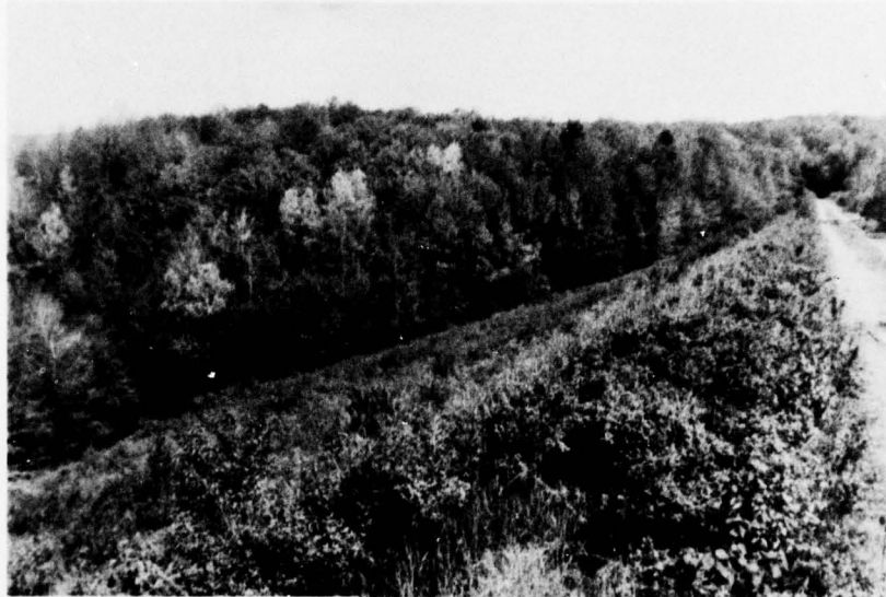
A. Embankment at Right Abutment
