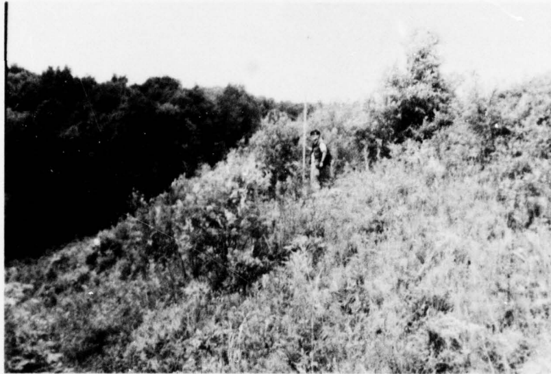
C. Brush on Downstream Slope of Embankment
