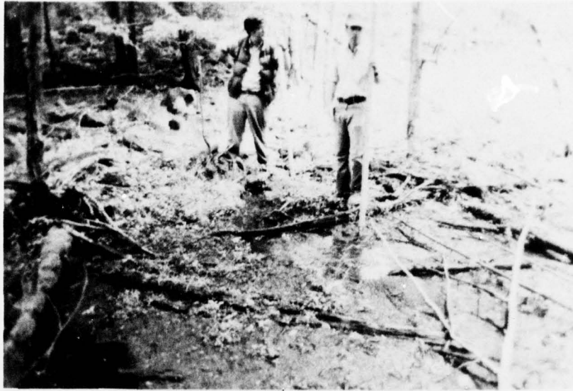
E. Seepage at Toe of Dam
