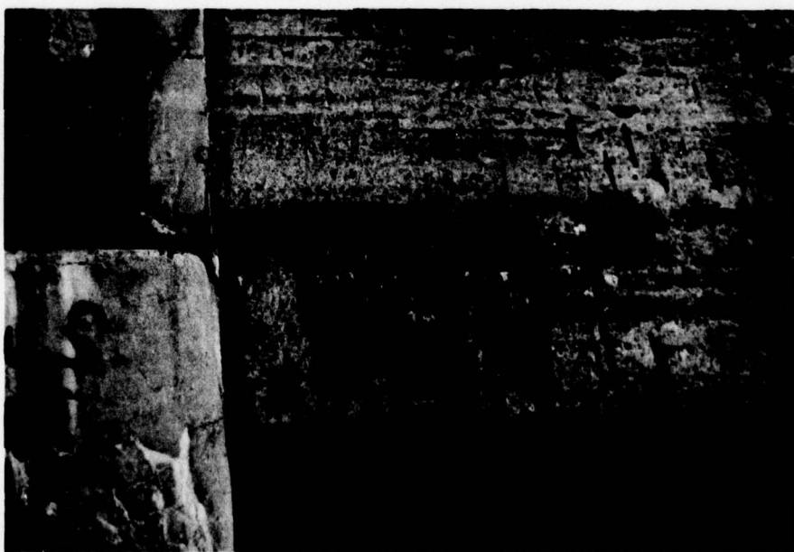
Seepage on Right Side Downstream Face of Spillway
