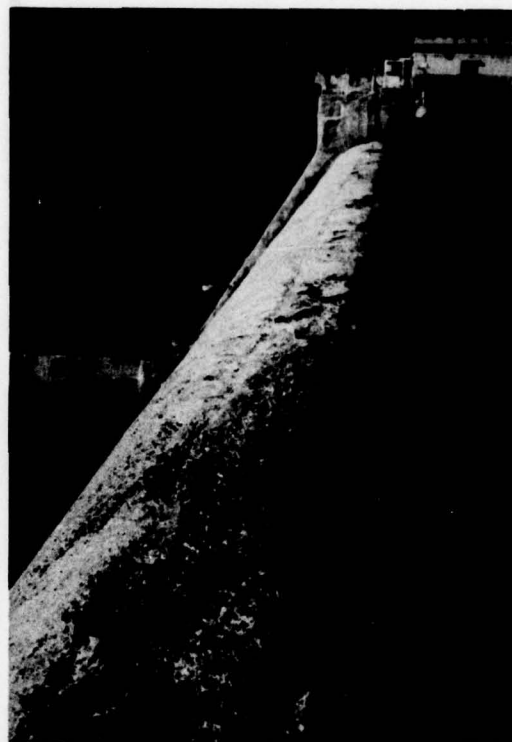
Concrete Deterioration of Face of Overflow Section. Note plugged 48" By-pass on Right Wingwall.
