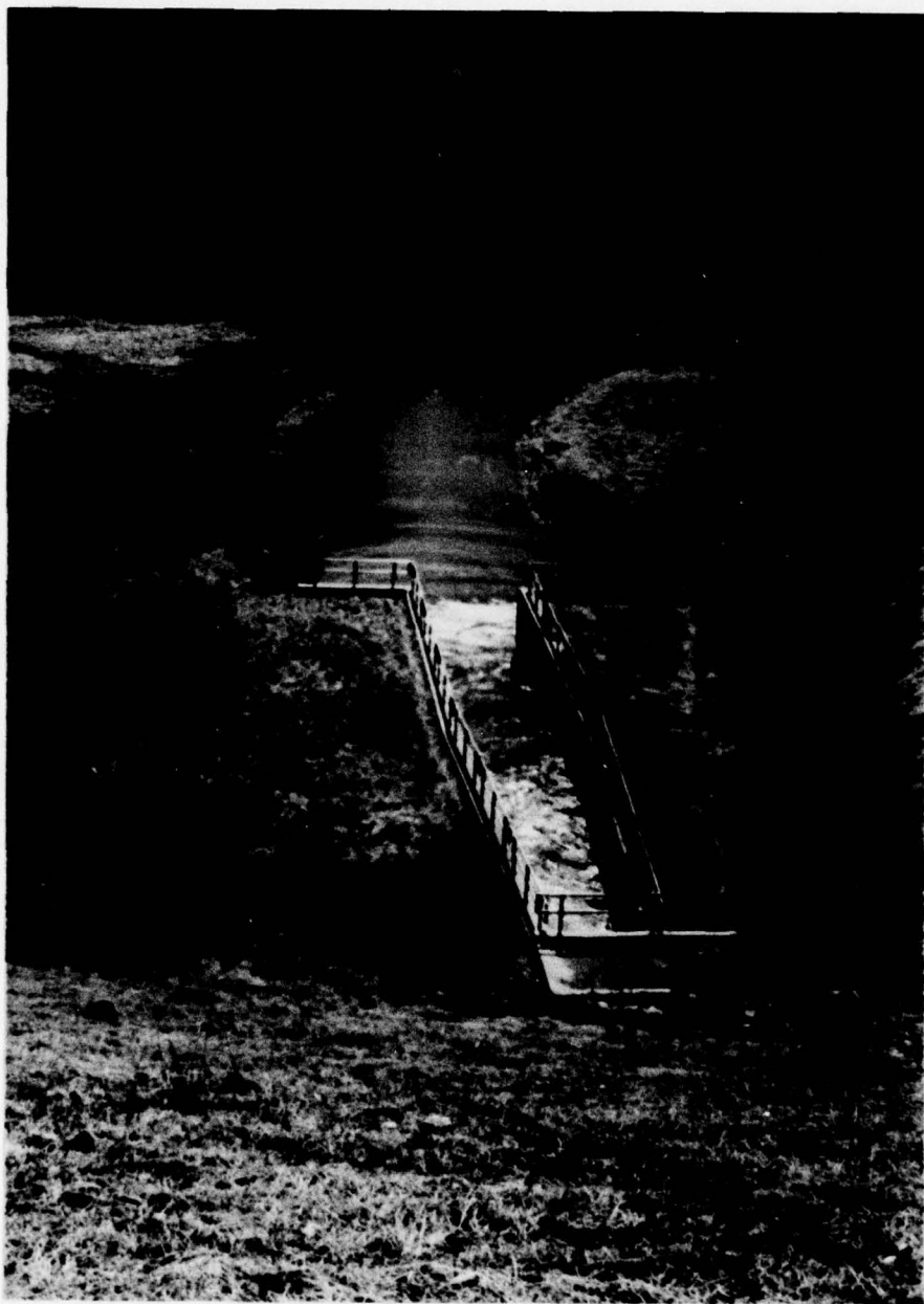
VIEW OF STILLING BASIN AND OUTLET CHANNEL WHICH CONTAINS DISCHARGES FROM THE PRIMARY SPILLWAY AND CONTROL TOWER.
