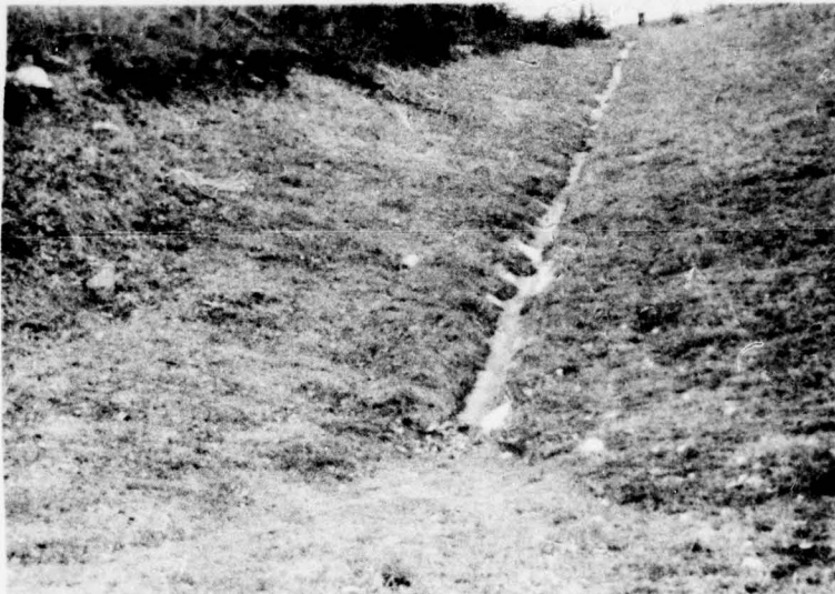
Right Concrete Gutter
