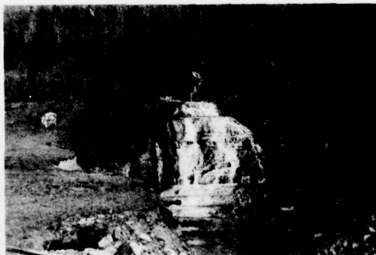
VIEW OF DAM OUTLET CHANNEL. NOTE SCOUR FROM FLOOD OF JULY, 1977
