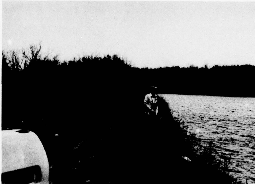
I. Olyphant No. 3 Dam Located Upstream of Olyphant No. 2 Dam View from Left Abutment
