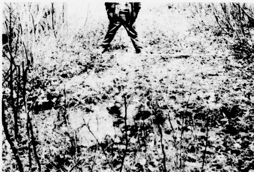
F. Wet Area at Left of Spillway Apron
