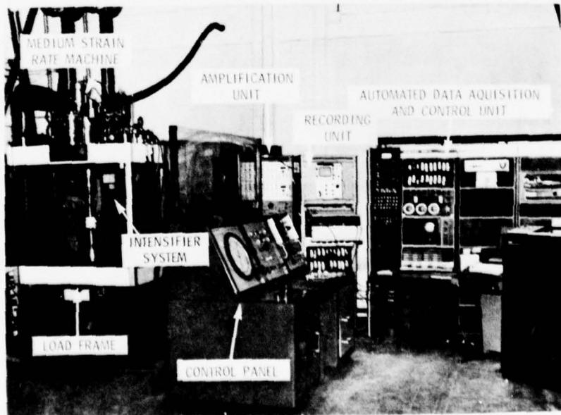
Figure 1. Automated materials characterization system.
