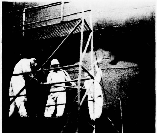
Figure 10 Photographs of the GLACIER During the Application of Inerta 160 (Upper) and Zebron (Lower)
