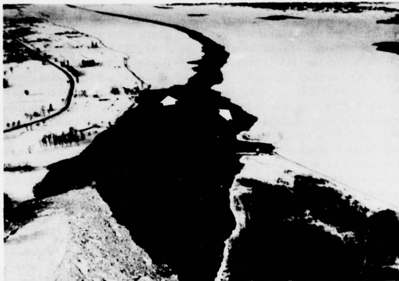
Figure 3. Head of Little Rapids Cut showing ice cover behind west boom (upper left arrow) cracked free from shore. Right arrow indicates east boom.
