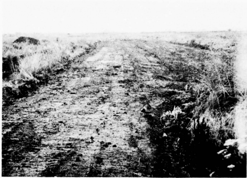
a. Mounded subgrade for interior haul roads was constructed with the small wide-track dozer. Material was bladed from the right of the photograph and semicompacted to form the haul road pad shown in the center of the photograph
