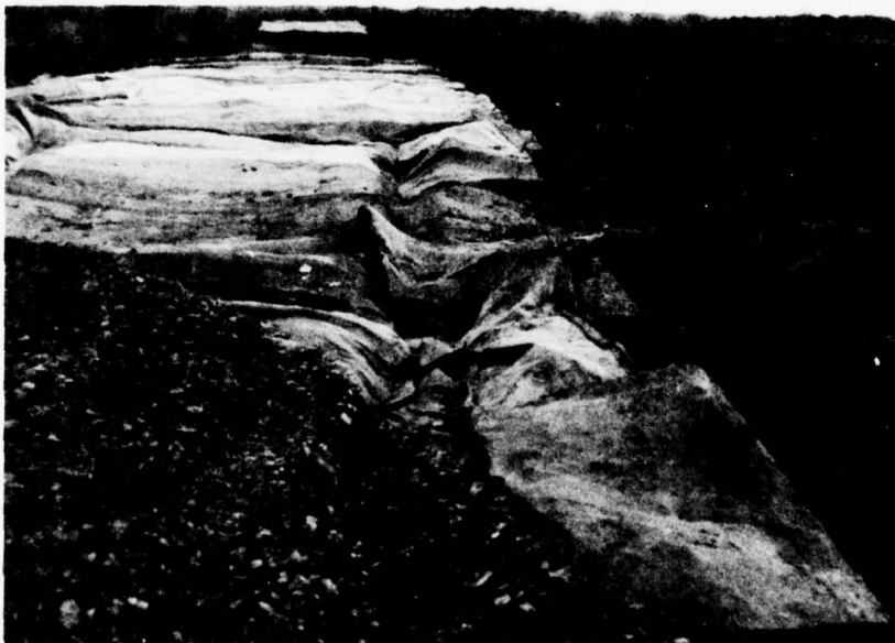
Figure 10. Rutting in the fabric-supported subgrade occurred when trucks backing down the haul road spreading shell continued to back after their load was exhausted. The photograph illustrates the need for fabric cover to obtain desired roadway performance
