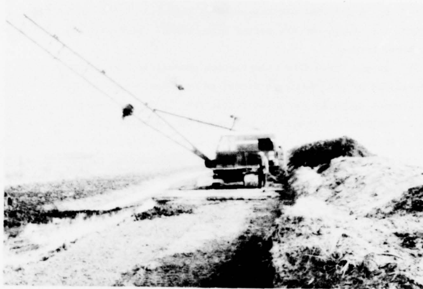
Figure 16. Large dragline shown removing crust from inside perimeter of east dike. Crust bench under dragline mats will be used for construction of second lift. Note mounds of borrow along alignment placed by previous truck haulage from interior borrow area. Small dragline is shown in background placing second lift in long partial segment construction
