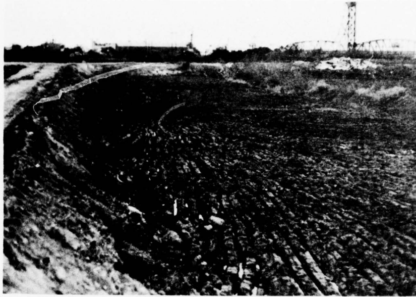
Figure 13. View along edge of spur haul road after dredged material crust had been removed. No evidence of subgrade bulging, foundation bearing failure, or mud waves is seen in the photograph
