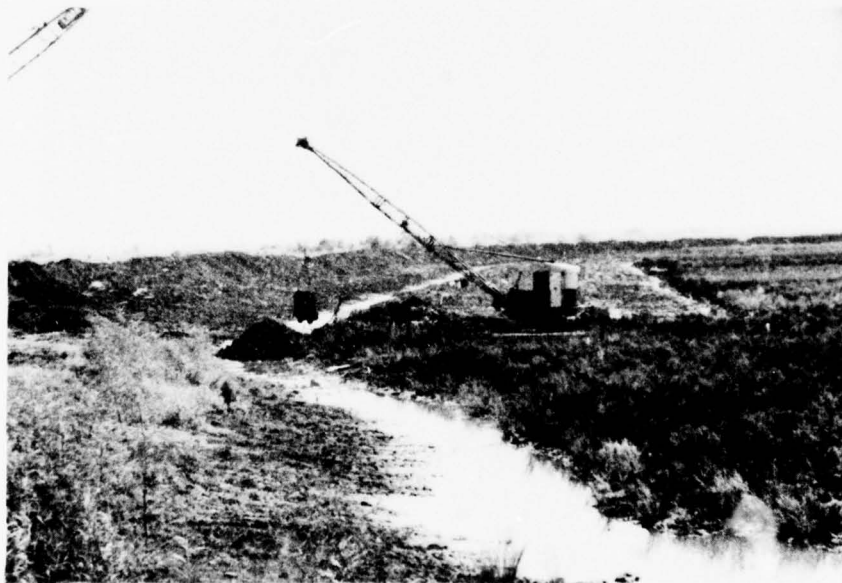
b. View of small dragline working on mats inside perimeter dike. Note pile of material placed for large dragline rehandling and drainage ditch maintained after borrow removal
