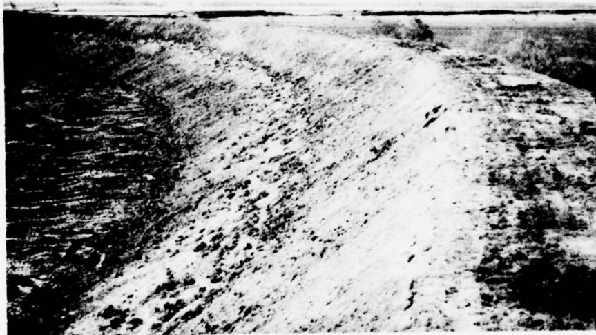
b. View of the completed raised perimeter dike
