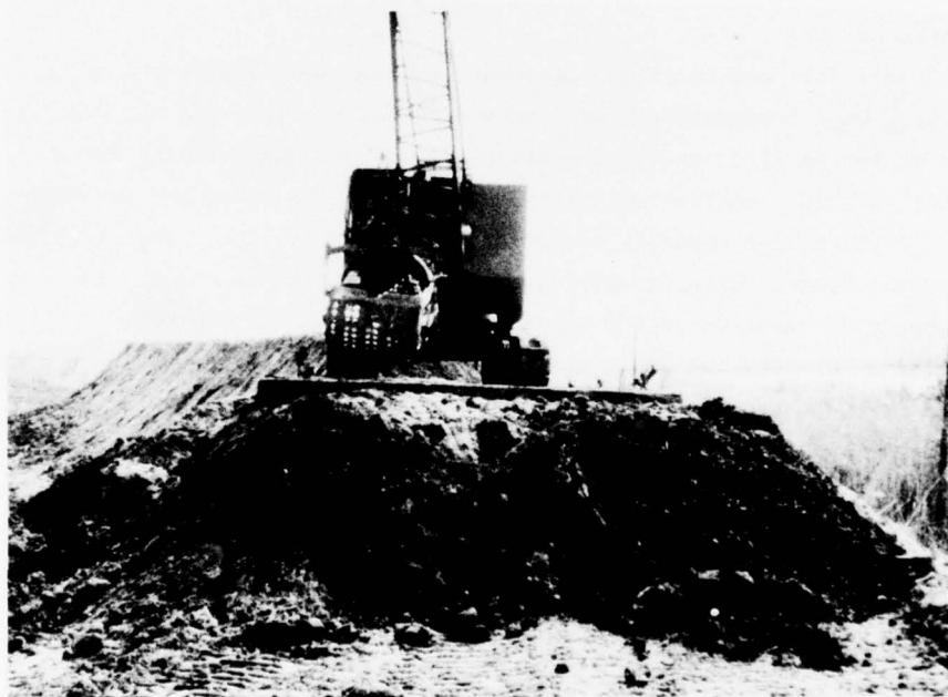
Figure 19. In the sequential dike construction technique, the dragline constructs the first lift ahead for a short distance, then rotates its boom and constructs the second lift behind, while moving down the dike alignment
