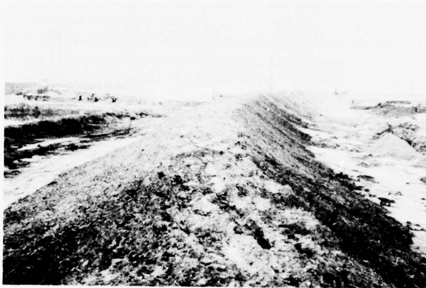
Figure 22. Dike segment of essentially coarse-grained material constructed between east dike and DOP underdrainage experiment location. View looking east from the east dike toward the DOP underdrainage experiment. Note traces of snow on the embankment
