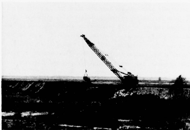
b. After initial construction, the second lift was placed and crest and side slopes dressed by the dragline
