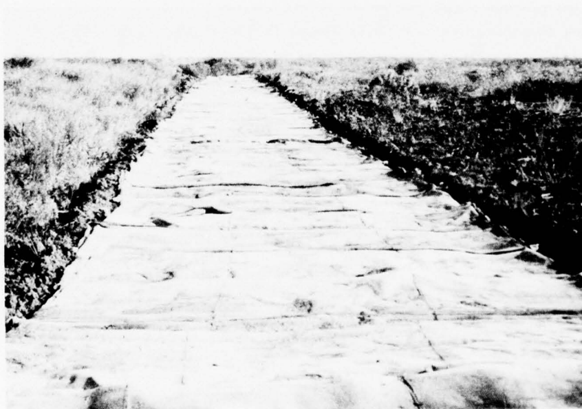
b. After the pad was complete, 12-ft-square sheets of filter fabric were laid on the pad and overlapped
