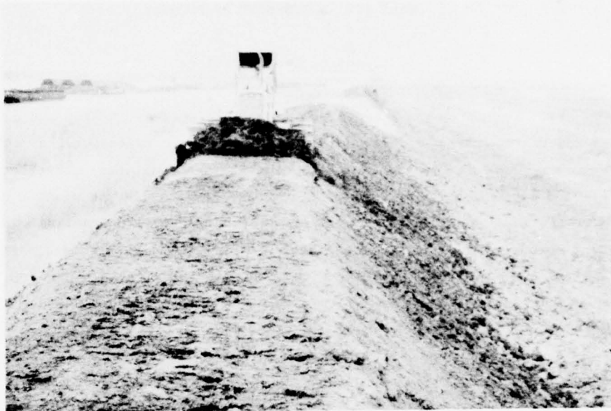
a. As the last construction operation, the small wide-track dozer bladed the dike to 8-ft crest width at El. 24 MSL
