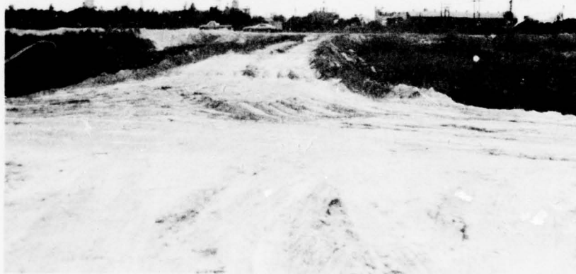
b. Condition of cement waste surface on spur haul road after approximately 400 load repetitions
