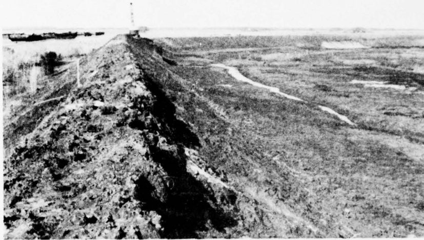
Figure 20. Rain-induced sloughing and sliding of uncompacted second lift. Note rotational slumping on inside slope with crest subsidence. Underlying semicompacted first lift was not affected
