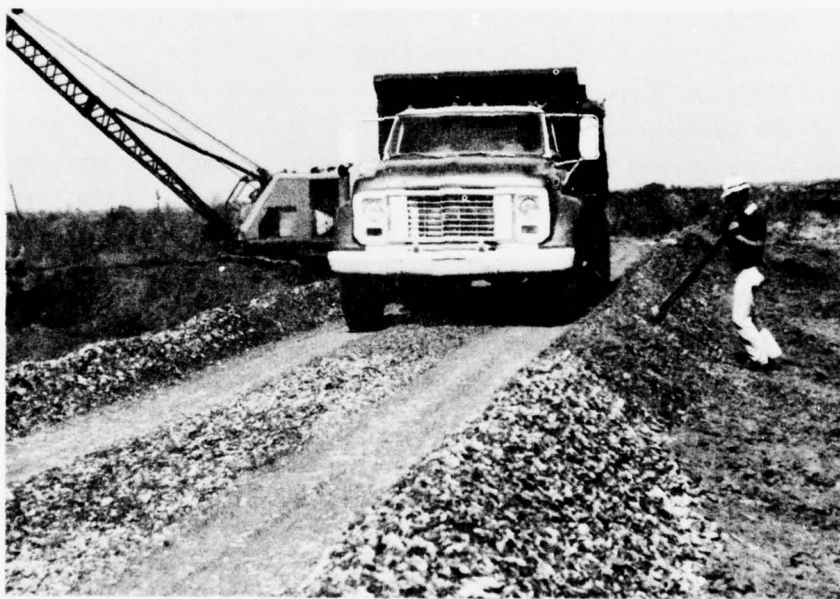
Figure 12. Photograph of spur haul road surface after approximately 300 load repetitions. Note relatively good condition of surface with minimal rutting in wheel paths
