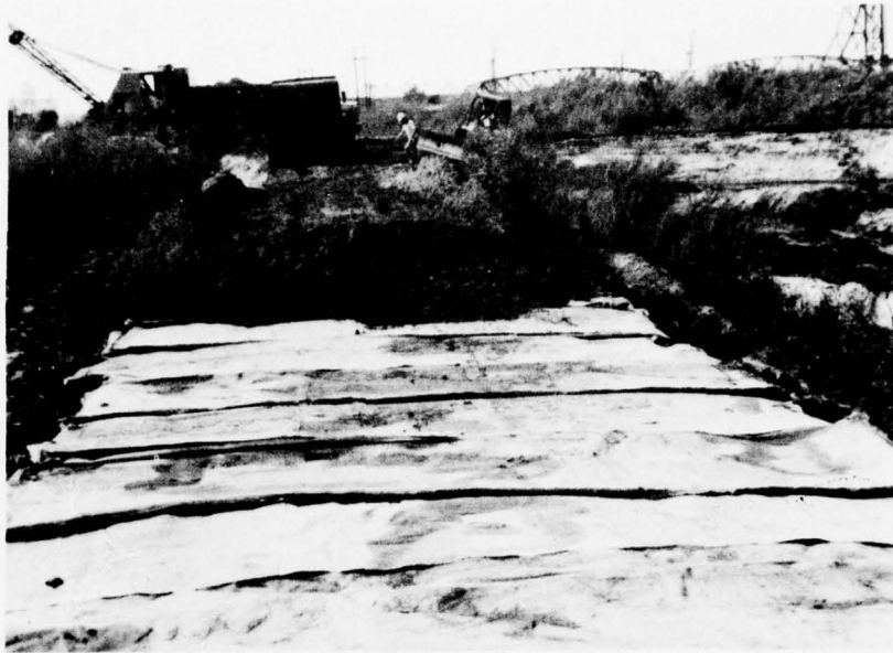
a. Cement waste evaluated as road surfacing is shown being placed on the fabric-covered subgrade. Note the resemblance of the partially hydrated cement waste to sand
