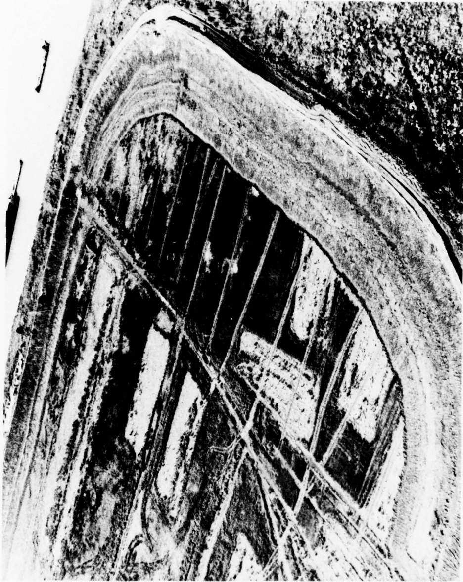
Figure 7. Aerial view of north end of Upper Polecat Bay Disposal Area, looking west southwest from northeast corner. Note strip of dewatered fine-grained dredged material removed around disposal site perimeter
