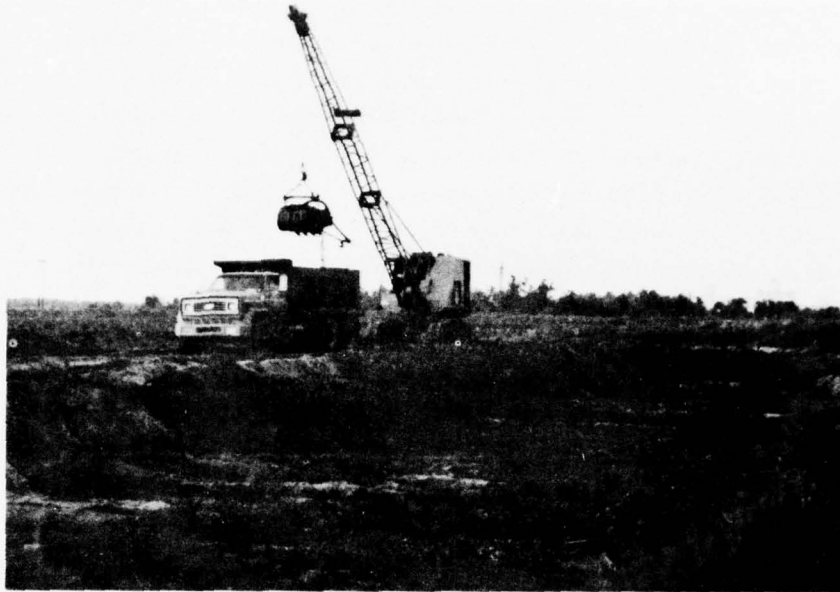
Figure 11. Medium dragline shown loading dump trucks with dewatered fine-grained dredged material in interior borrow area
