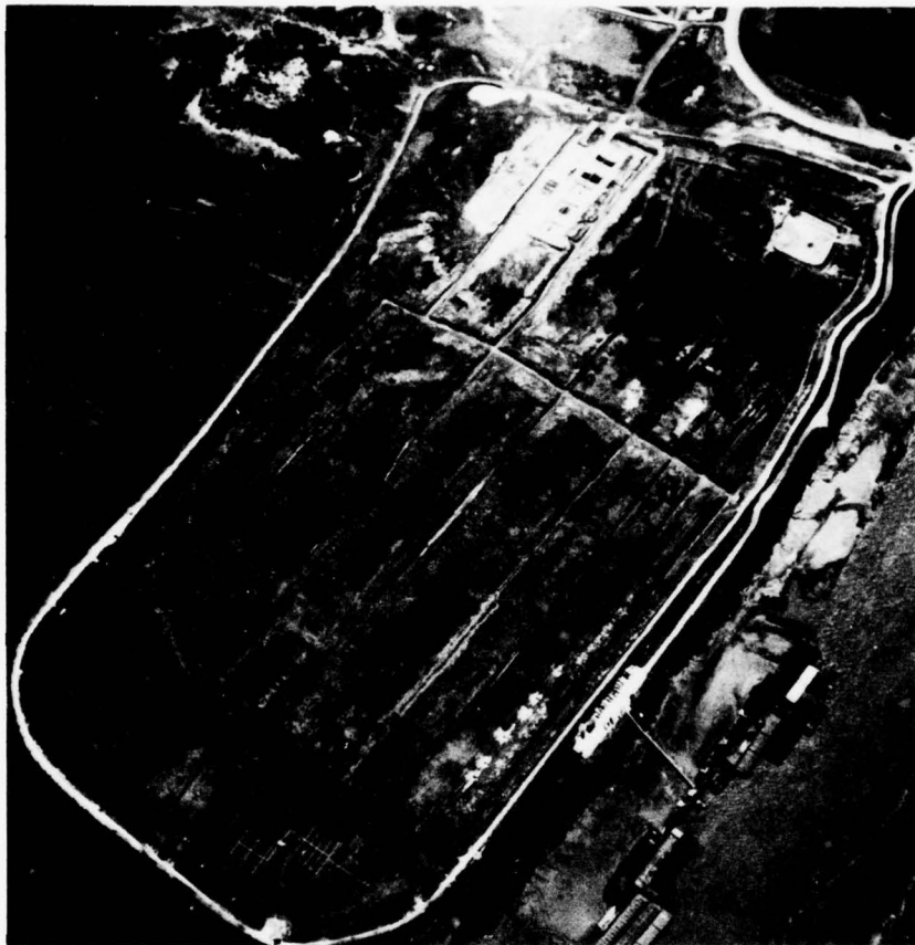
Figure 2. Aerial view of Upper Polecat Bay Disposal Area prior to initiation of dike-raising activities. Note the surface drainage network produced by DMRP DOP dewatering field demonstrations. North toward the lower left corner of the photograph
