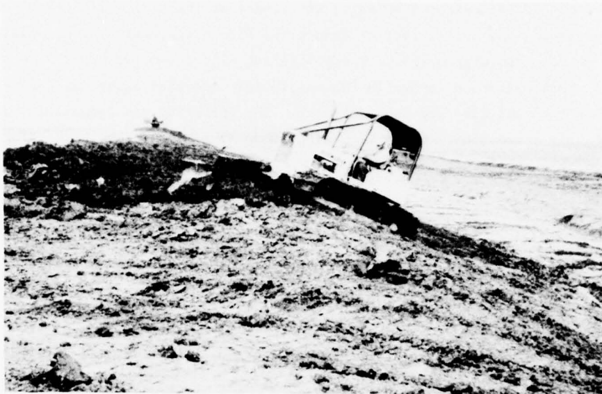
Figure 18. Small wide-track dozer shown constructing first lift while dragline in background of photograph constructs second lift and dresses the crest and side slopes
