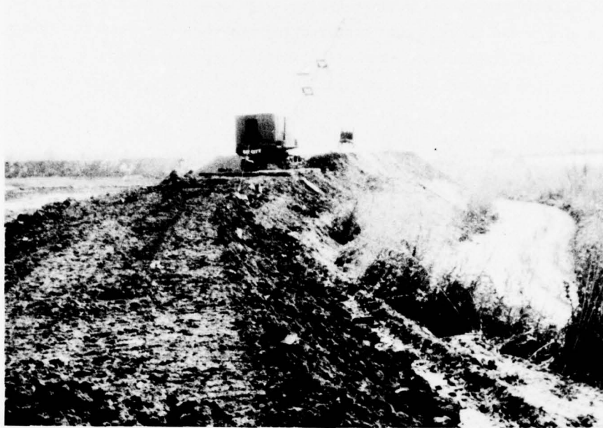
a. Dragline is shown completing first lift along east dike. Borrow in foreground has been roughly shaped by dozer to facilitate precipitation runoff. Ragging on stake in center of photograph indicates El. 20 MSL, crest elevation for first raise lift
