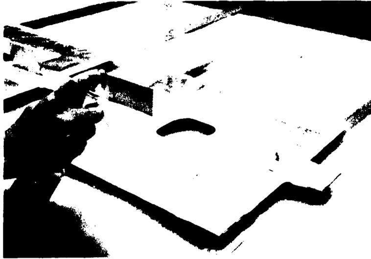
*Figure 23. - Priming Surface with BR127 Primer*
