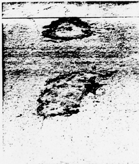
FIGURE 6.14 FINISHED REPAIR OF AREAS 3 AND 4
