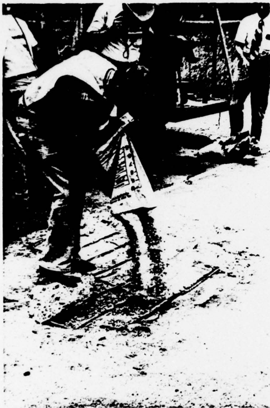
FIGURE 6.9 DRY AGGREGATE ADDED TO AREA 1
