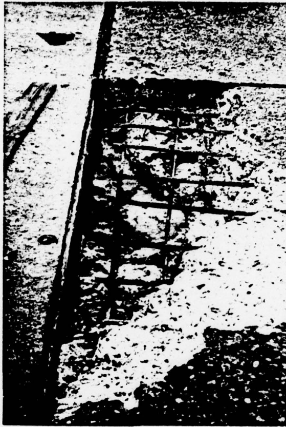
FIGURE 6.3 REPAIR AREA 1 AFTER REMOVAL OF CONCRETE
