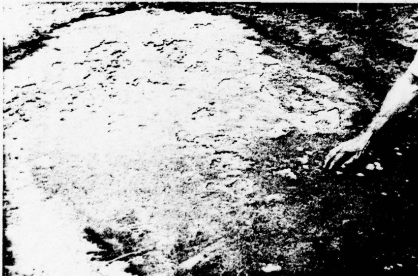
FIGURE 6.12 BLISTERING OF AREA 1
