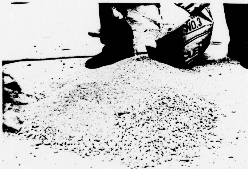
FIGURE 6.23 MIXING OF SAND AND 3/8-IN. TOPPING ROCK
