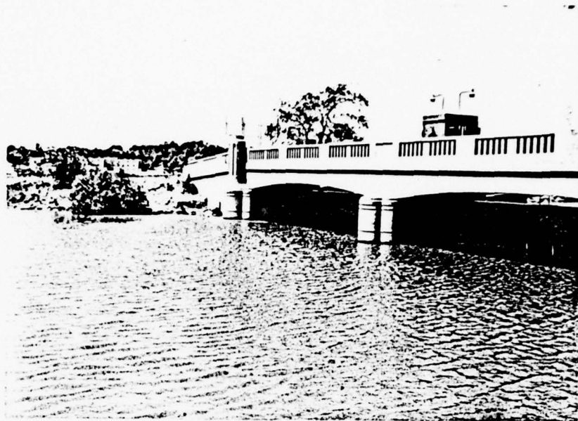
Upstream view of Structure June 1978
