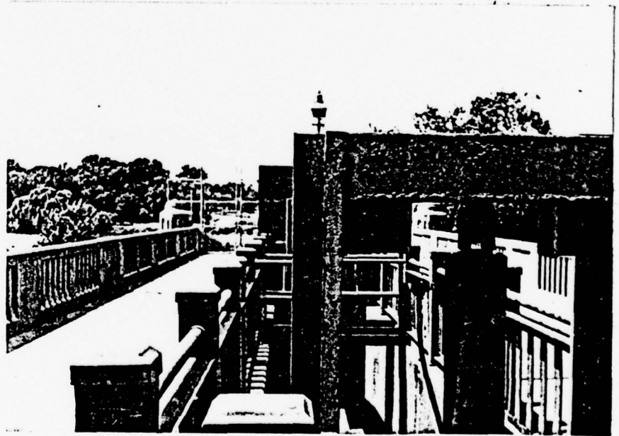
Lifting Apparatus July 1978
