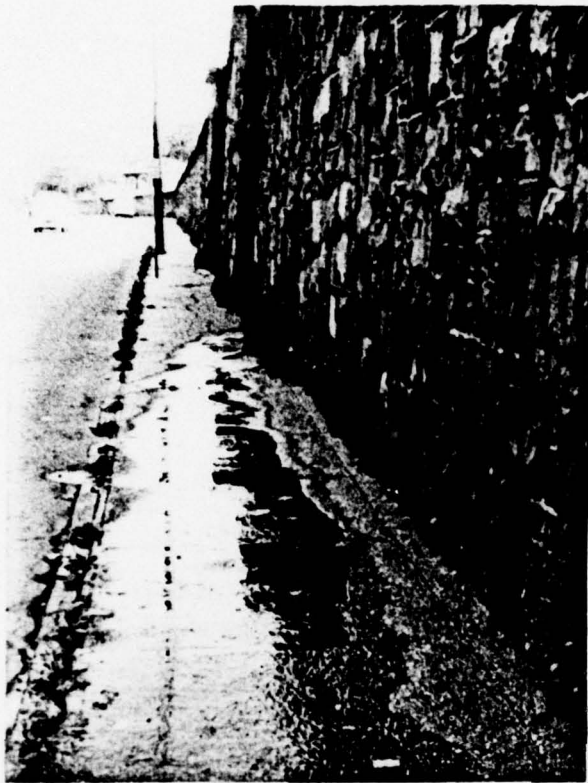
LEAK AT WEST WALL
