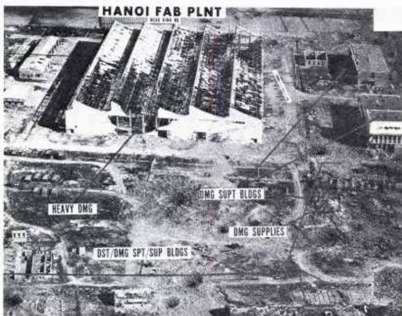
Hanoi Fab Plant
