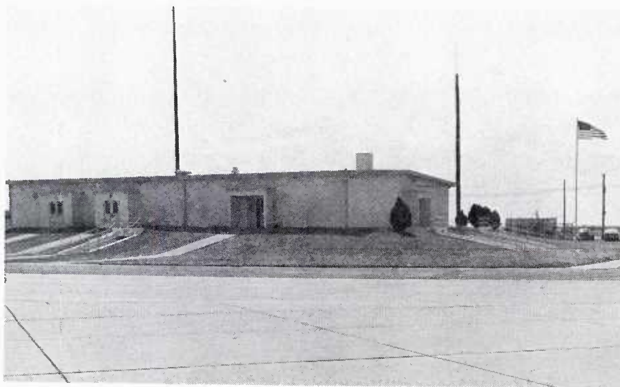
Satellite base facility
