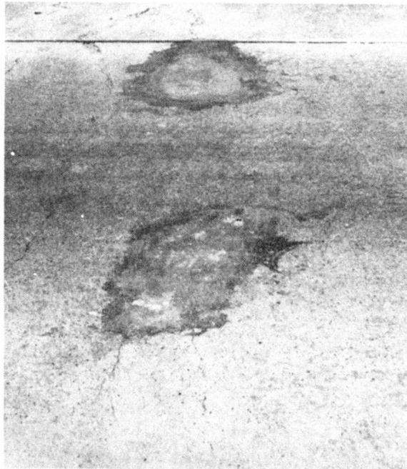
Figure 51. Finished Repair of Areas 3 and 4
