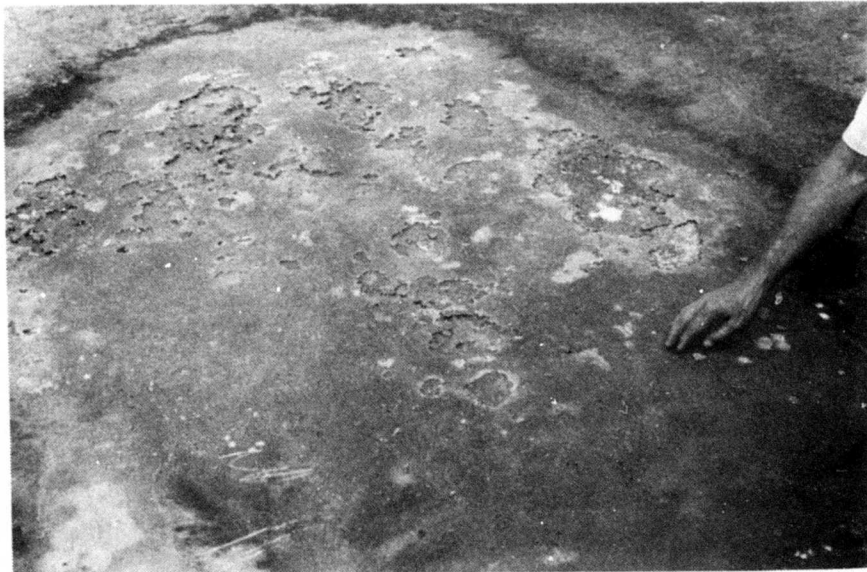
Figure 49. Screed Finish on Area 5
