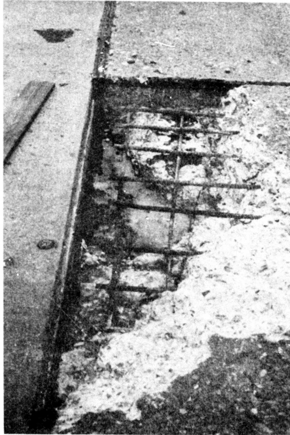
Figure 40. Repair Area 1 After Removal of Concrete
