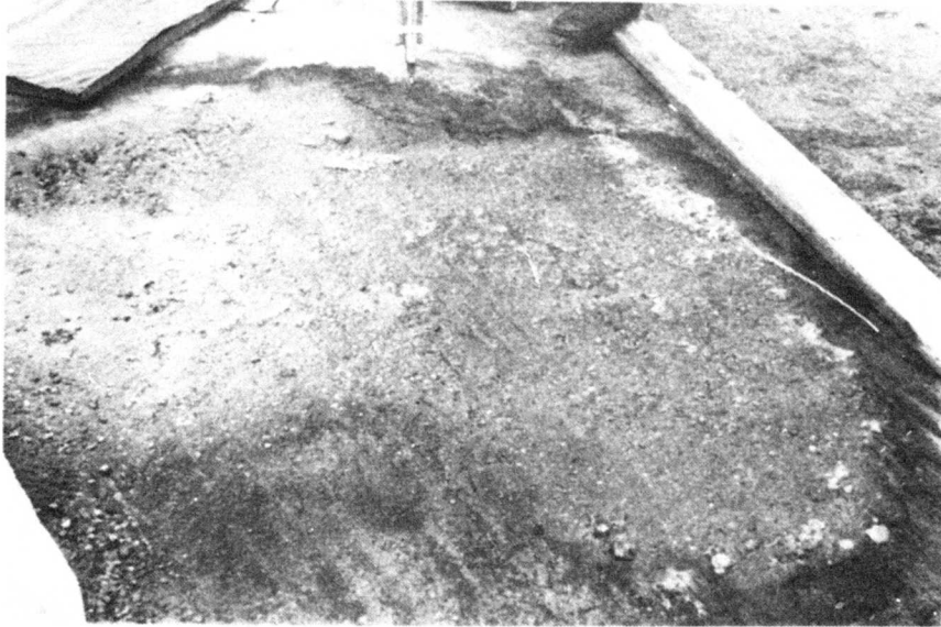
Figure 50. Blistering of Area 1
