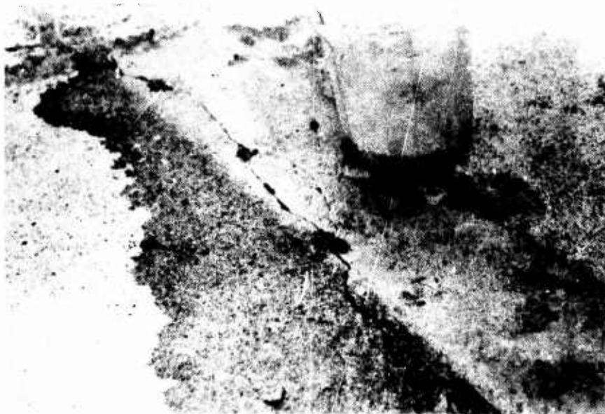
Figure 64. Saturating Area 4 with Monomer
