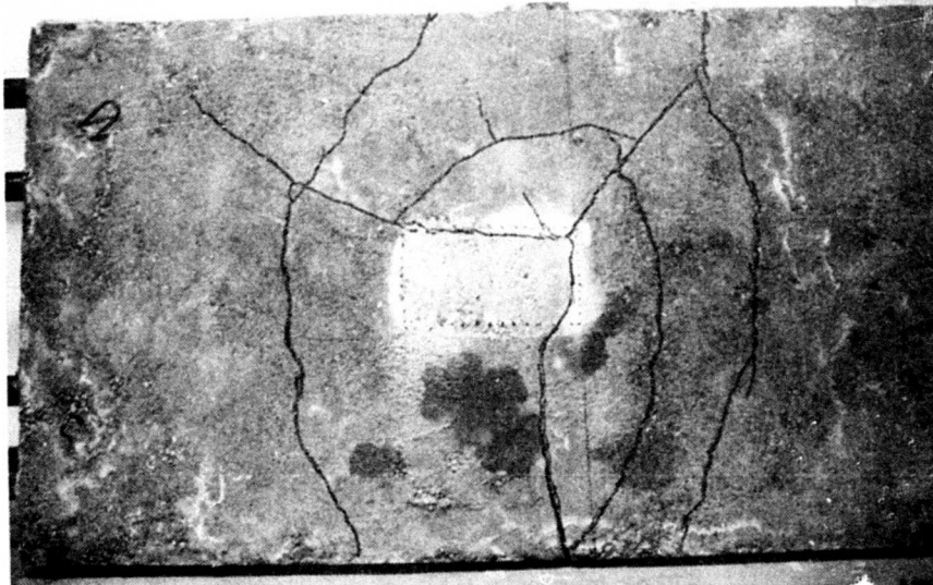
Figure 32. Top of Slab 2
