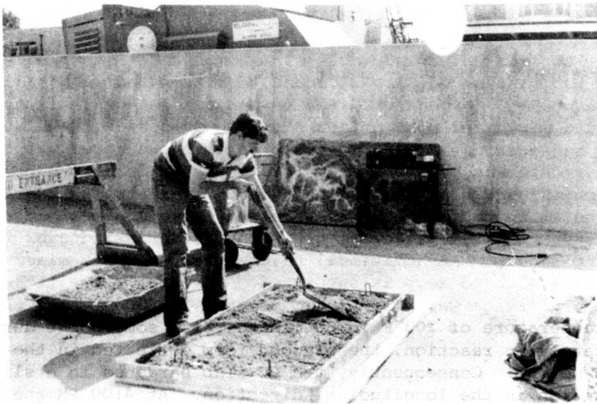
Figure 27. Slab 2 Being Poured
