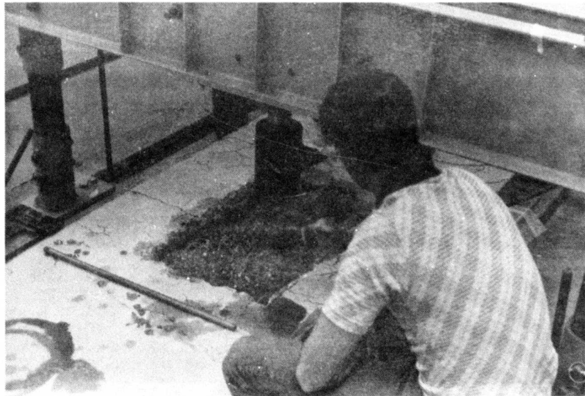
Figure 24. Slab 1 With Concrete Removed
