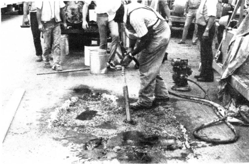
Figure 48. Vibration of PC: Area 1
