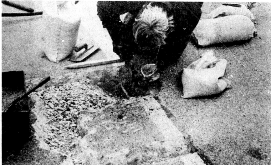
Figure 41. Repair Area 3 Interstate Highway 35
