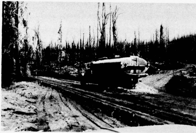
FIG. 15.--WATERING IS NECESSARY TO MINIMIZE DUST PROBLEMS ON FEEDER ROADS
