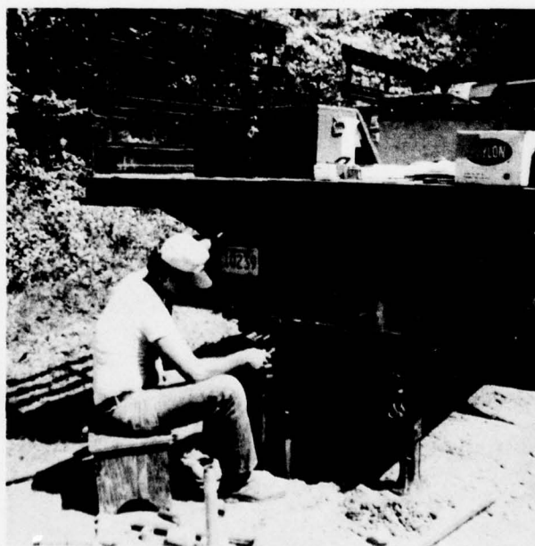
FIG. 4.--CALIFORNIA BEARING RATIO MEASUREMENT IN PROGRESS ON A LAYER OF A TEST SECTION
