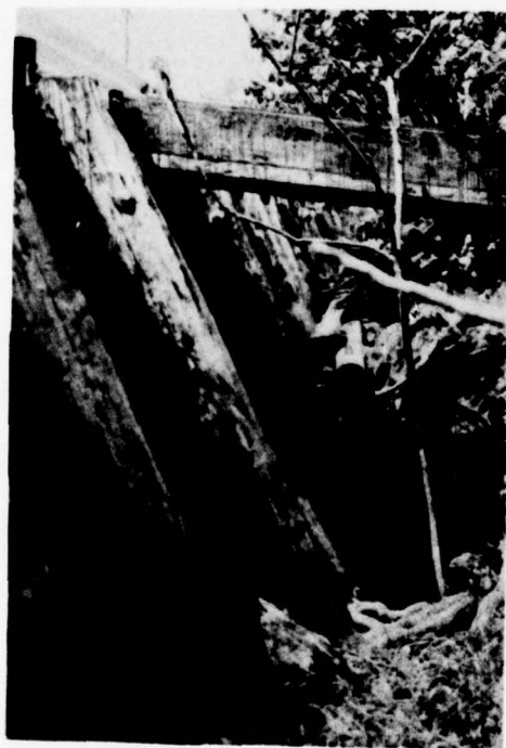
Photo 12 - Close-up of the downstream timber pile supported retaining wall; the wood structure visible at the top of the wall is a roadway drainage trough
