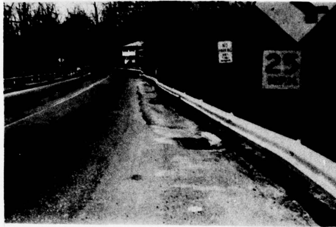
Photo 9 - View of the roadway forming the dam crest, looking toward the left abutment; the guardrail on the downstream face has moved with the timber pile supported downstream retaining wall; the roadway paving has cracks paralleling the dam axis, also indicating downstream movement
