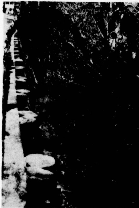
Photo 9 - View of the roadway forming the dam crest, looking toward the left abutment; the guardrail on the downstream face has moved with the timber pile supported downstream retaining wall; the roadway paving has cracks paralleling the dam axis, also indicating downstream movement
