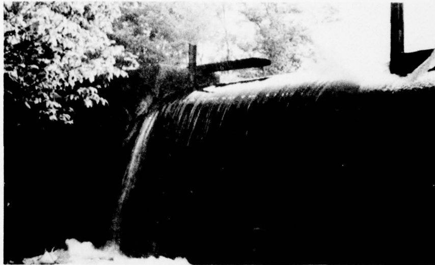
SPILLWAY WITH ONE FLASHBOARD
